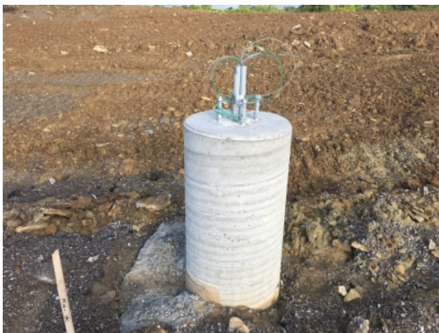
2018.08.21 – Installed light pole base.
