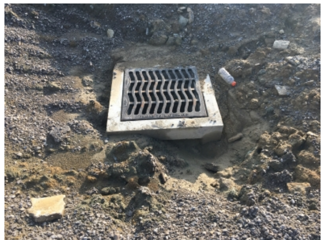
2018.08.21 – Storm structure missing erosion control measures.
