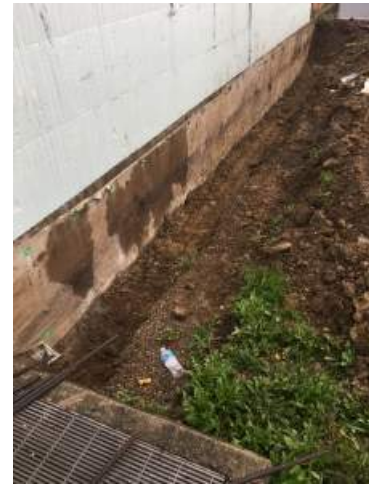
2018.08.08 – Excavation for new brick ledge.
