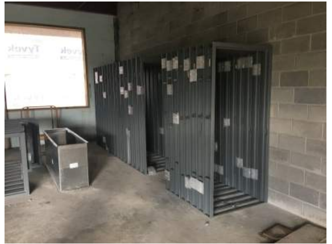
2018.08.21 – Hollow metal frames staged for installation.
