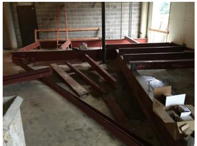
2018.08.08 – Band corridor ramp framing.
