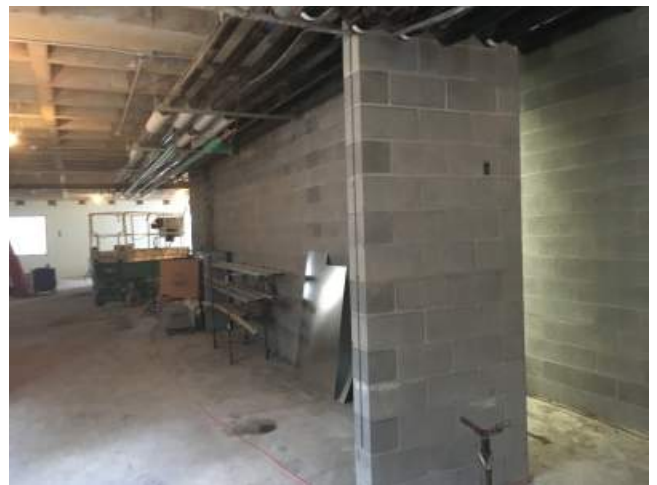
2018.08.21 – Masonry wall @ electrical/mechanical room.
