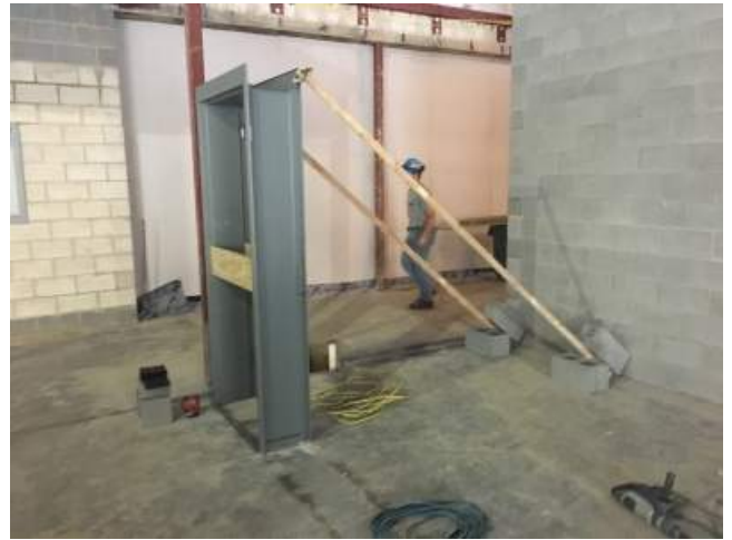
2018.08.21 – Door frame set and braced.
