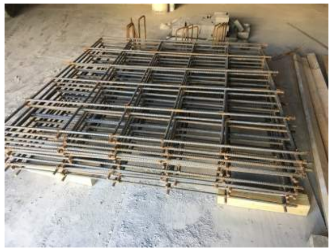
2018.08.28 – Reinforcing for shade structure footings.
