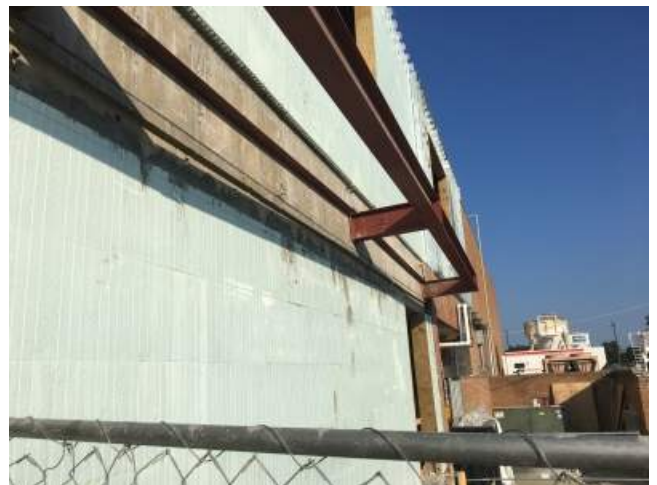
2018.08.28 – Steel framing at canopy.
