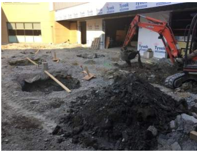
2018.08.28 – Shade structure footing excavation.
