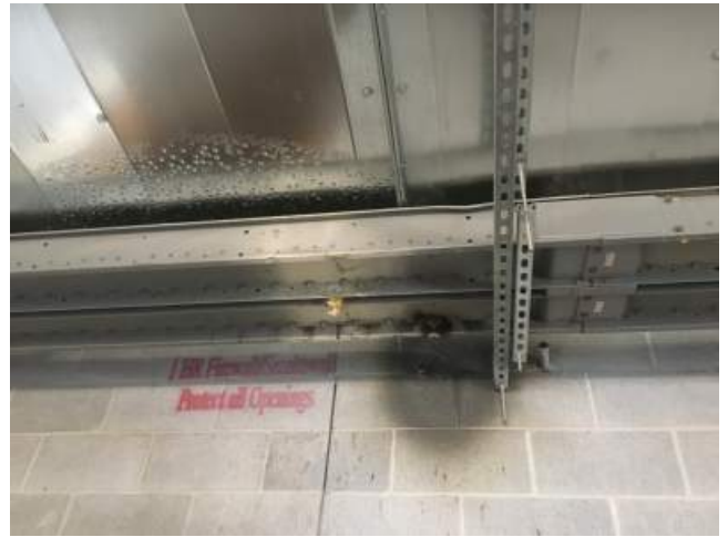
2018.08.22 – Failed electric bus duct.
