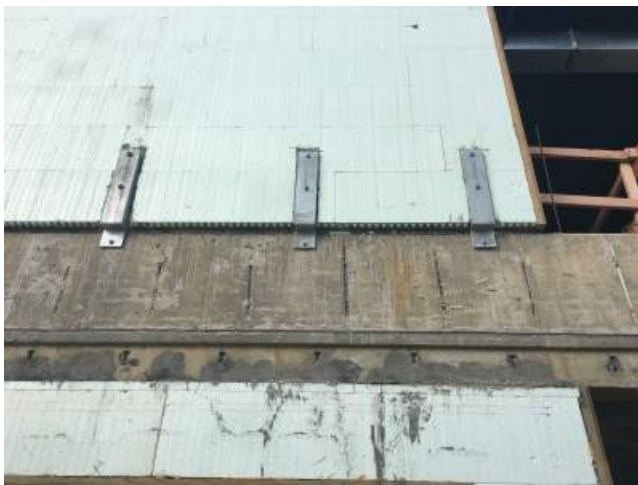
2018.08.21 – Steel channel supports for brick ledge.
