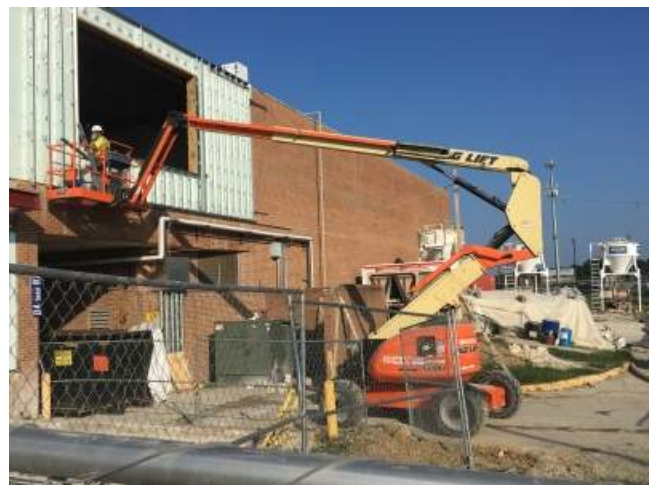
2018.08.28 – Installation of exterior furring.
