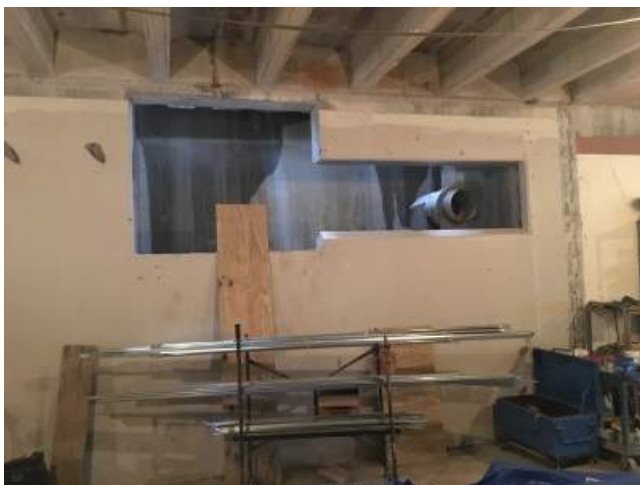
2018.08.08 – New opening into area well.
