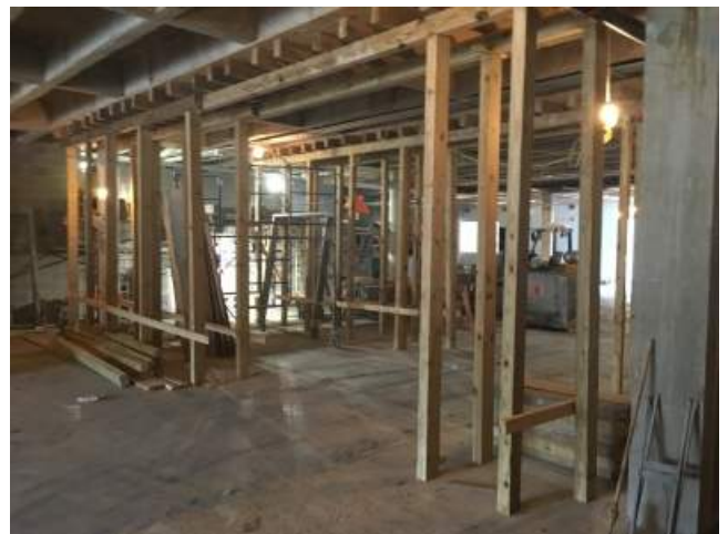
2018.08.21 – Shoring under new slab reinforcing.
