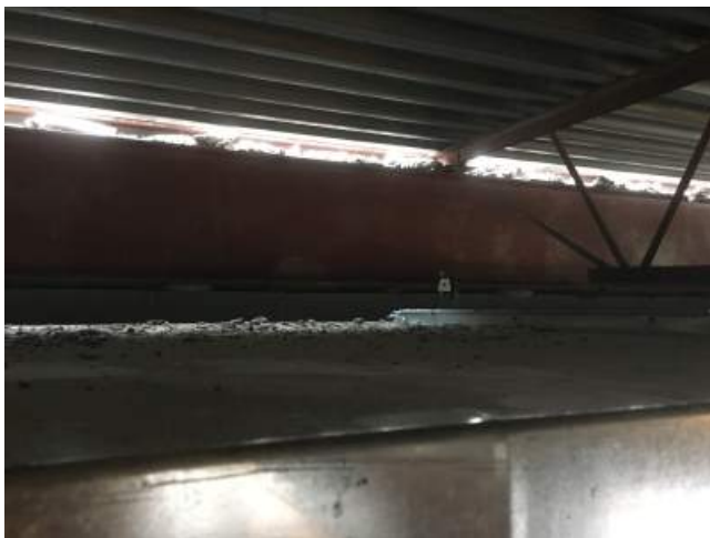
2018.08.22 – Daylight visible at wall above failure.
