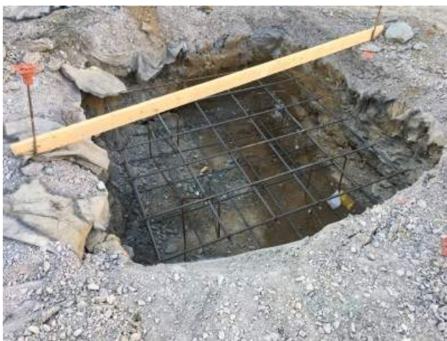
2018.08.28 – Shade structure footing prepared.
