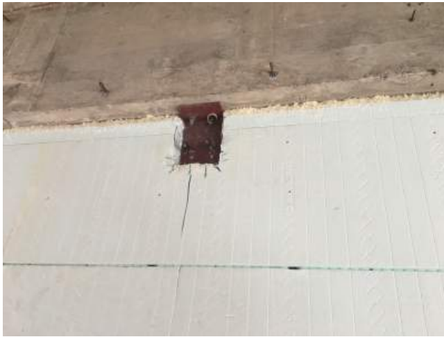
2018.08.21 – Lateral bracing at ICF along Lonneman.
