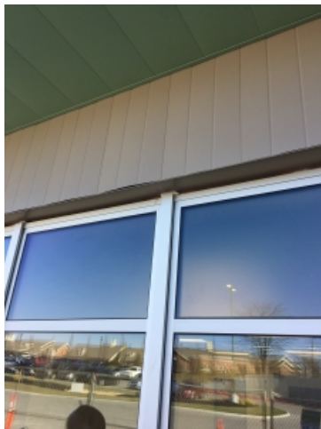
2018.03.12 – Unacceptable undulation at siding.
