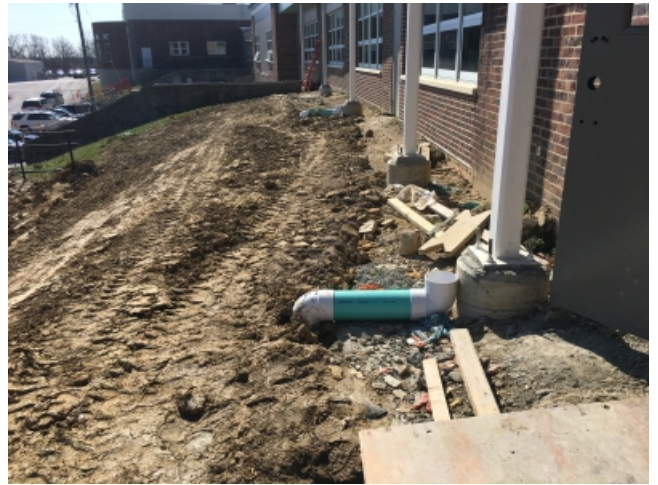
2018.03.12 – Downspout collector at East elevation.
