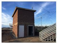
Items to complete include the storage room doors, fascia cover, handrail, second-level guard wall, ceiling, and hardware installed, the interior finished and cleaned, electrical completed, and asphalt patched around the exterior.
