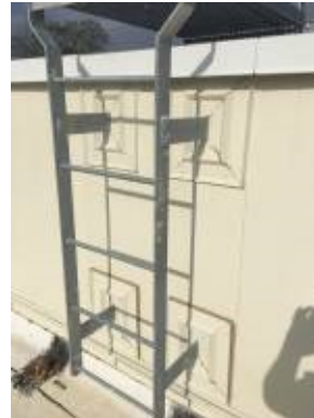
2017.10.12 – Proper ladder installation at new gym wall panels
