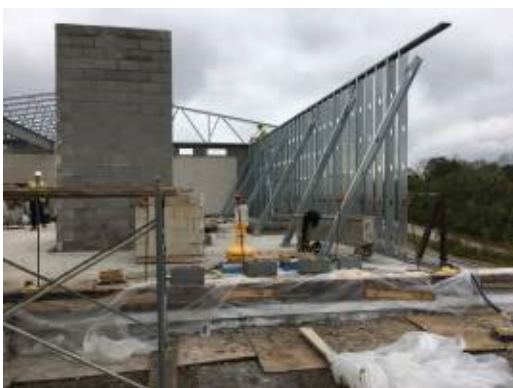
2017.10.12 – Stud framing and completed elevator shaft
