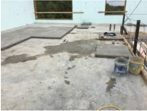
2017.10.12 – Housekeeping pads at 2 nd floor
