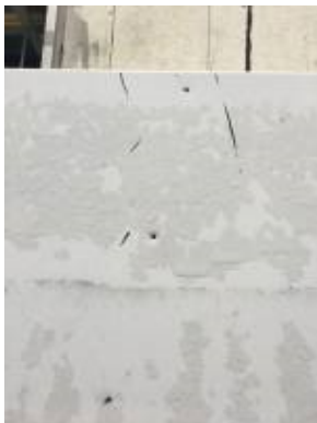
2017.10.12 – Holes in exg coping potentially allowing water into new wall insulation
