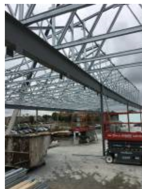
2017.10.12 – Installed roof trusses
