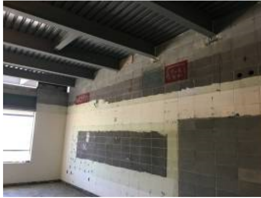
2017.09.28 – Layout of duct penetrations at existing classroom wall
