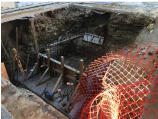
2017.09.28 – Formwork and reinforcing at west end of basement stairs
