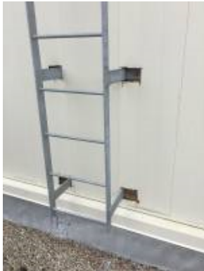
2017.10.12 – Improper ladder installation at new gym wall panels
