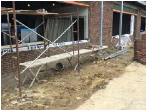
2017.10.12 – Brick infill below window opening in existing wall
