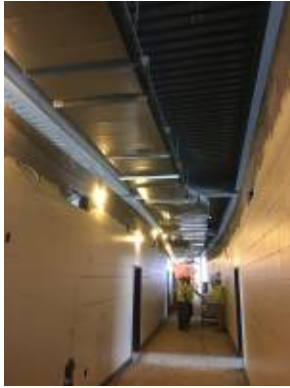
2017.09.28 – Ductwork installed in corridor
