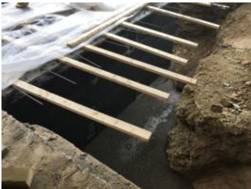
2017.10.05 – Flowable fill and waterproofing at basement stairs
