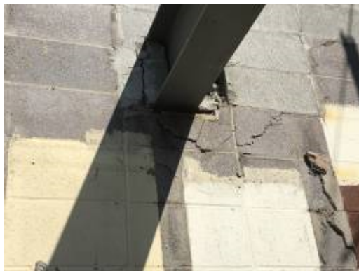
2017.09.28 – Damaged beam bearing to be repaired
