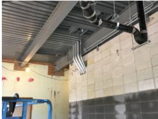
2017.10.12 – Conduit and plumbing below 2 nd floor mechanical room
