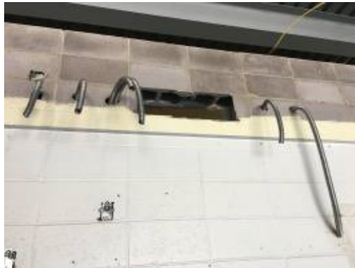
2017.09.28 – New electrical conduit in existing CMU classroom wall
