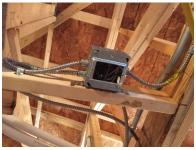
Conduit and mechanical lines are being run in the soccer building.
