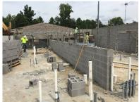
There is a lot of trash around the foundations of the buildings. This will need to be cleaned out before filling.
