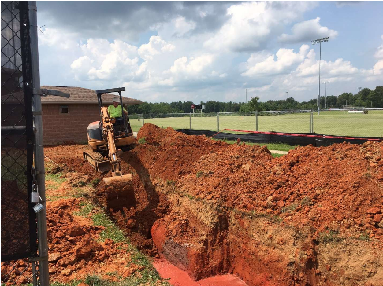
JHHS Soccer Building – Electric service excavation and encapsulation
