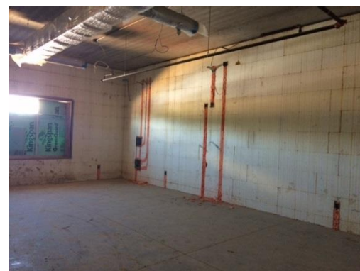
ICF walls, concrete planks above & concrete slab
