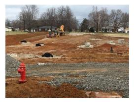
4. There are still some block masonry walls laid below the slab elevation that have not been grouted and are now accumulating trash and some have been filled with crushed stone. These need to have the trash removed and grouted up to the slab elevation.
