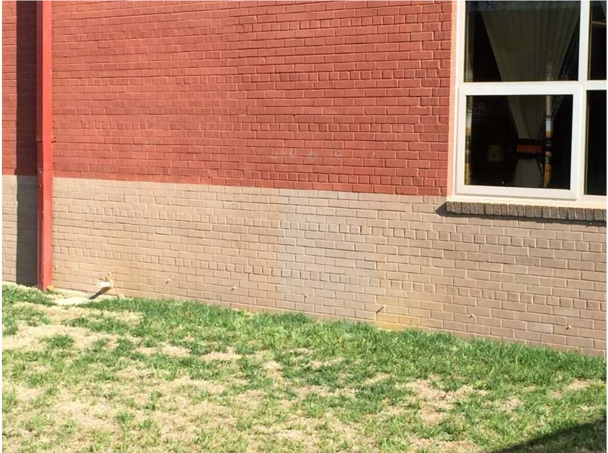
Image 2: West elevation following sealer application.
