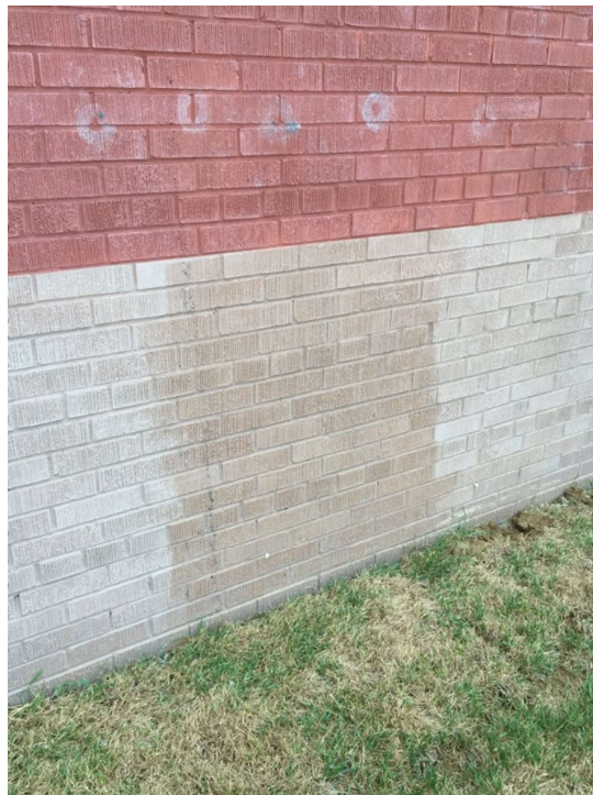
Image 1: Sample of sealer (prior to application at west elevation).
