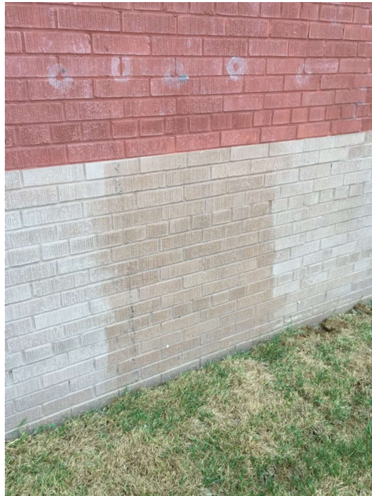
Image 2: Typical tuckpointing completed at the west elevation.
