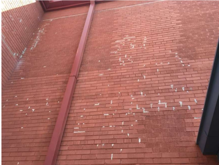
Image 2: Typical tuckpointing completed at the west elevation.
