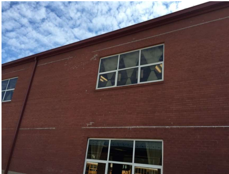
Image 1: Joints at head of infill previously completed were completely retooled and tuckpointed.
