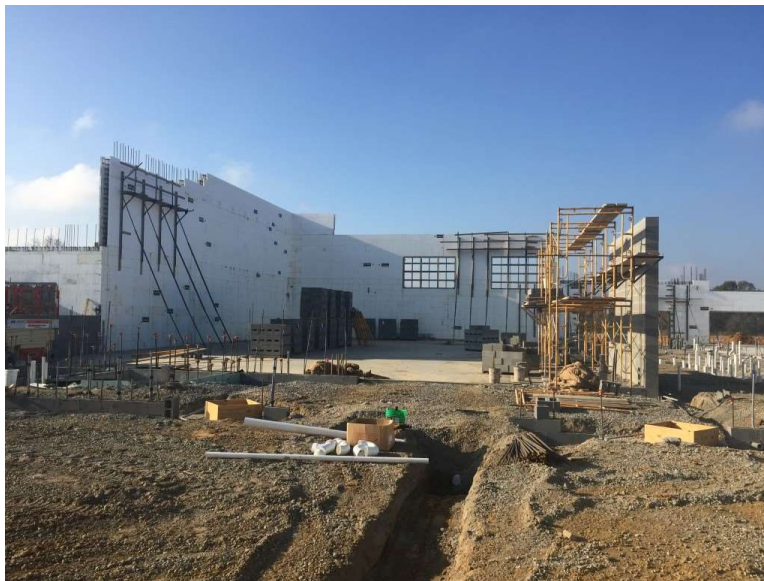
Photo 3: View of Gymnasium (beyond). Excavation is complete for CMU footings at Classroom demising walls (foreground).
