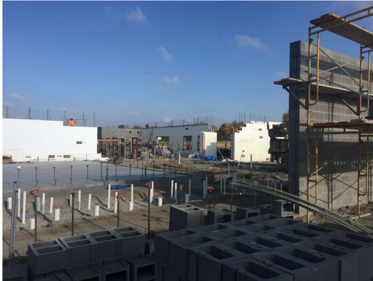
Photo 8: Masonry is ongoing at the first floor.
