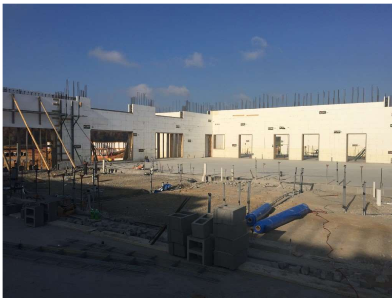
Photo 7: Cafeteria ICF walls are in progress. Floor slab at cafeteria has been poured.
