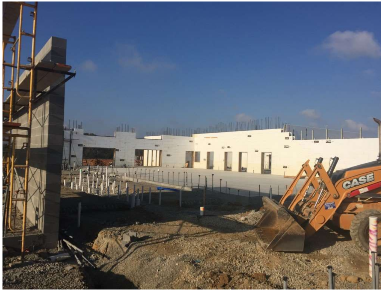
Photo 4: Wall footings and below slab plumbing are nearing completion at main first floor restroom bank (between Gymnasium and Cafeteria).
