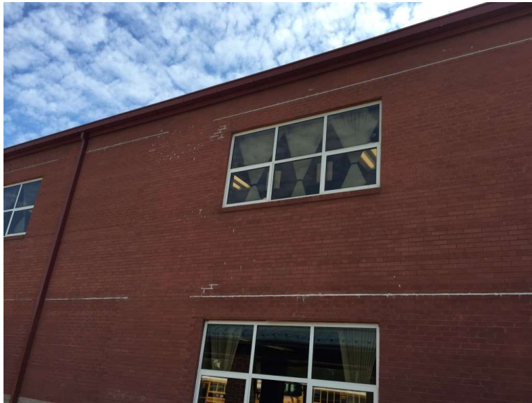
Image 1: Joints at head of infill previously completed were completely retooled and tuckpointed.
