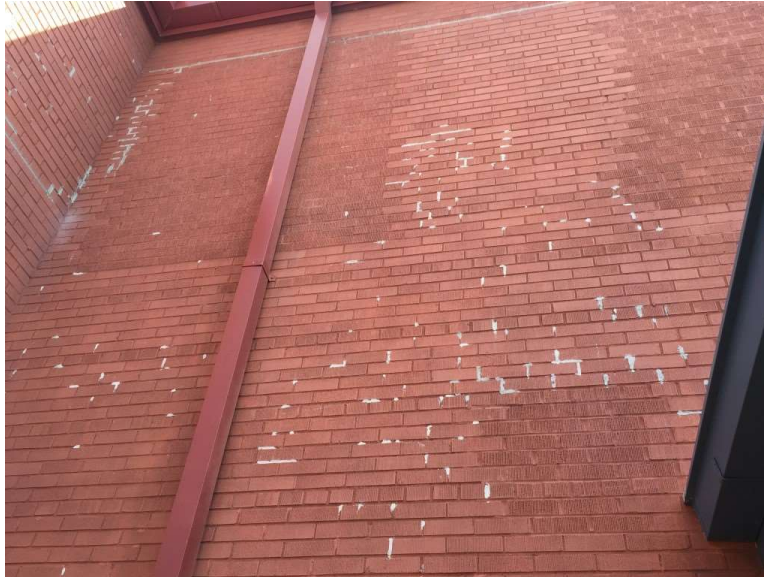
Image 2: Typical tuckpointing completed at the west elevation.
