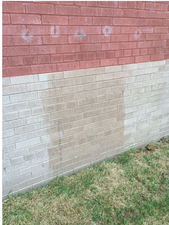
Image 2: Typical tuckpointing completed at the west elevation.
