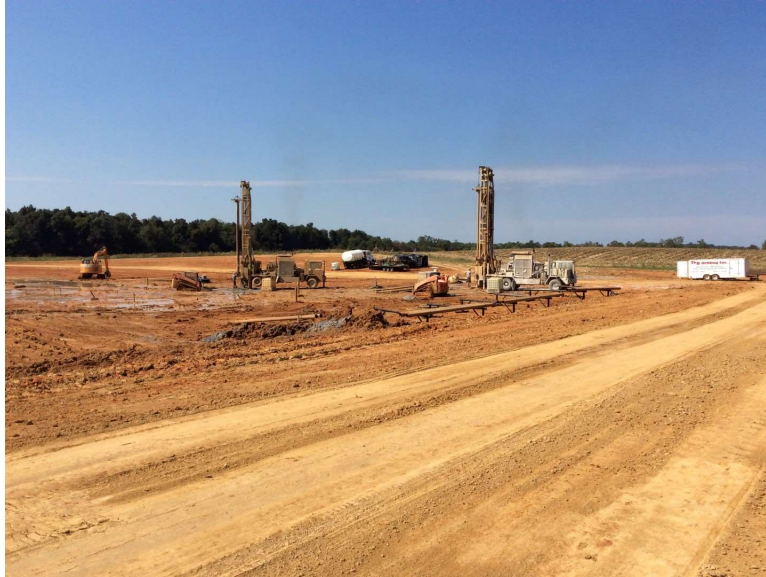
Photo 8: Geothermal wells are underway. Two (2) drill rigs are presently on site.
