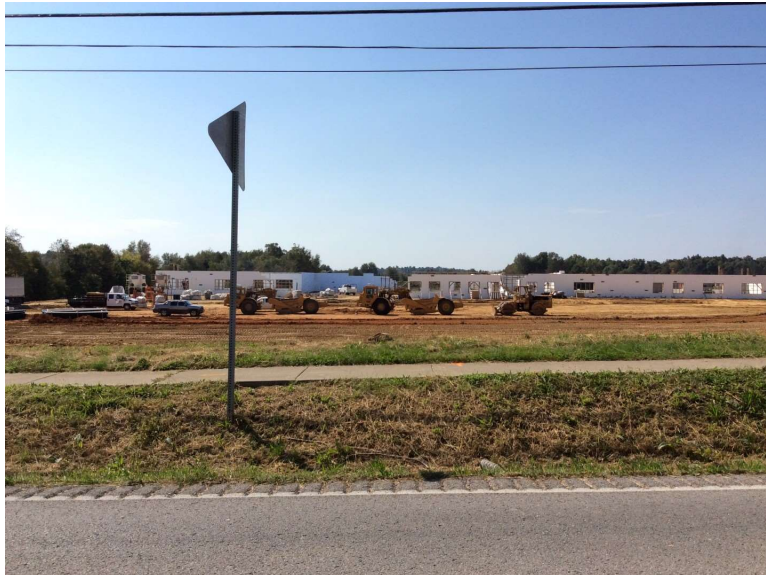
Photo 1: View from highway. ICF (Insulated Concrete Forms) continues at first floor.
