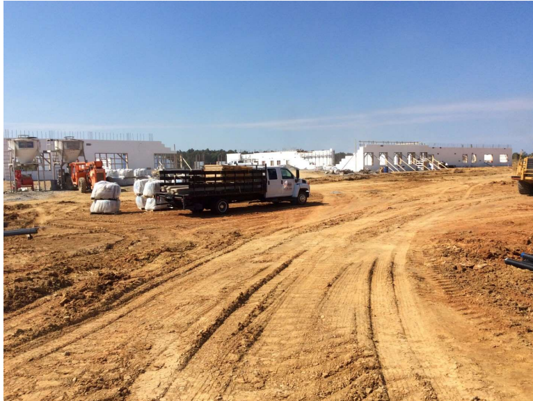
Photo 2: View of construction from the main entry.
