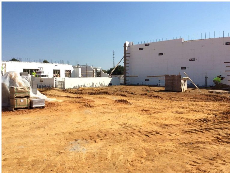
Photo 5: ICF exterior walls continue at the Media Center
