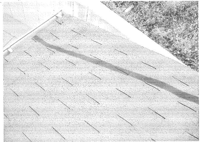
LOWER East Corner has water damage, deck under Shingles is Rotten And Needs Replacing.
