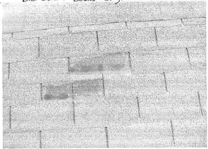
Shingle Roof old + Brittle, Several Tabs Broken
