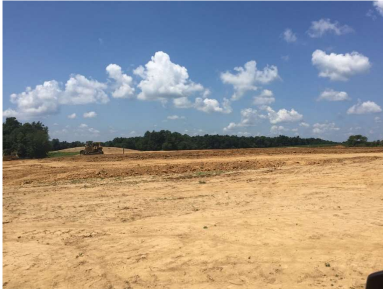
Photo 2: Building pad is being prepped in anticipation of beginning footings. GEM Engineering has reviewed site data to date and notified the Contractor that foundation excavations may be started (Photo 7/21/16).
