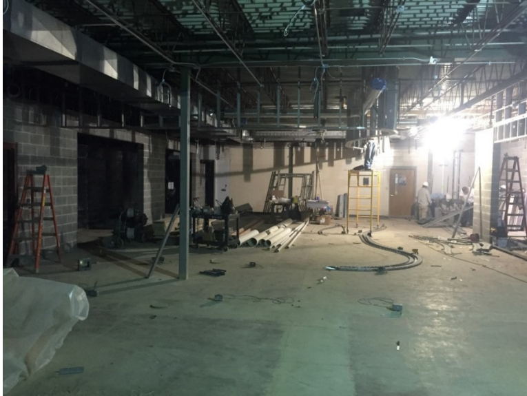
Image 5: Demolition is nearing completion in the new serving line area and kitchen. New soffits are being installed above future serving line locations.
