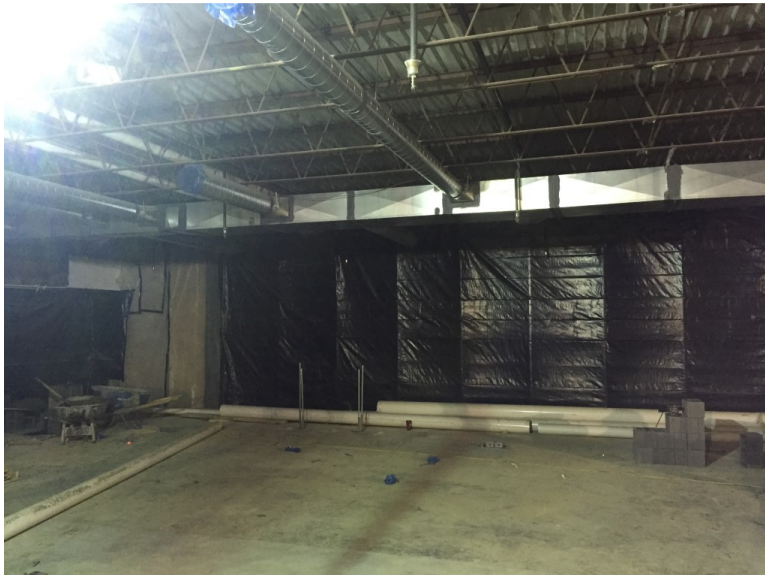
Photo 4: Temporary partition and dust protection separates occupied space from areas with ongoing construction.
