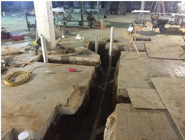
Photo 2: M/E/P rough-in below slab is ongoing at the kitchen
