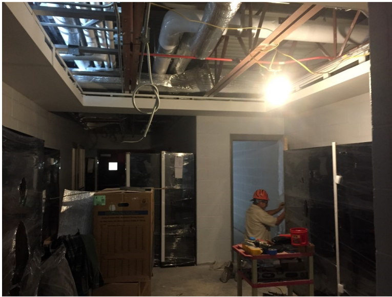
Photo 5: Mechanical rough-in is complete above ceiling at the existing locker rooms. Doors and hardware are being installed.
