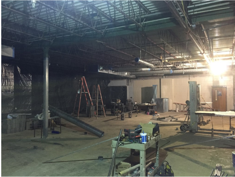
Photo 3: Mechanical rough-in above ceiling is ongoing at the new serving line and kitchen.
