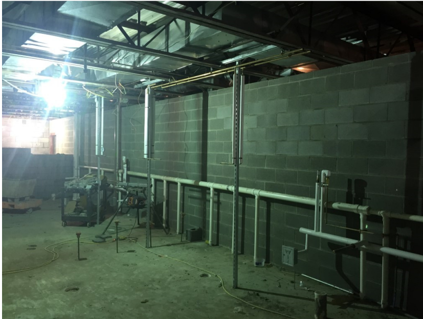
Photo 3: New mechanical, electrical, and plumbing systems rough-in is ongoing at the existing locker room area.
