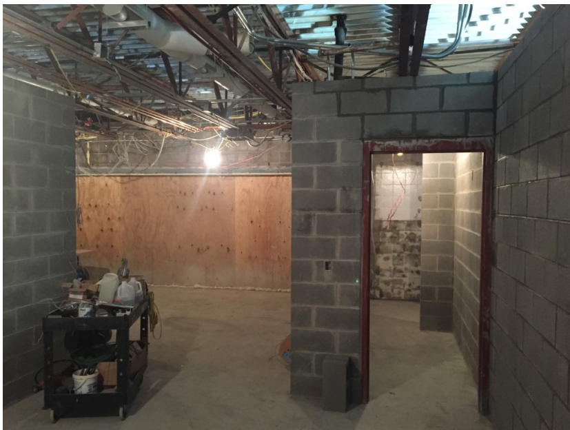
Photo 4: Floor slabs have been placed in the existing locker room area. Masonry is ongoing. Beyond, temporary partitions separate the existing gymnasium from the existing locker room area.
