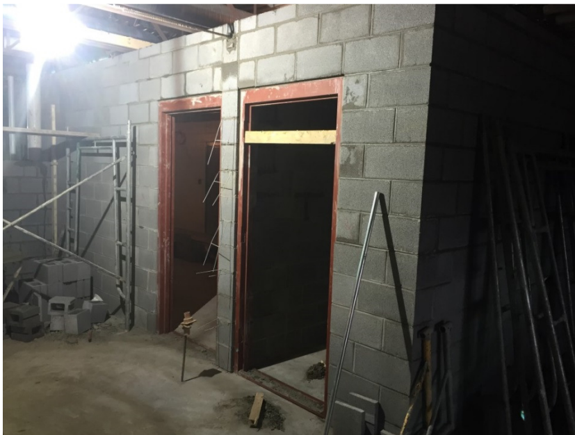
Photo 2: Hollow metal door frames are being set in the renovated existing locker room area.
