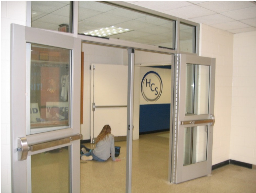
Photo 1: Storefront system and doors have been installed at the interior side of the security vestibule.
