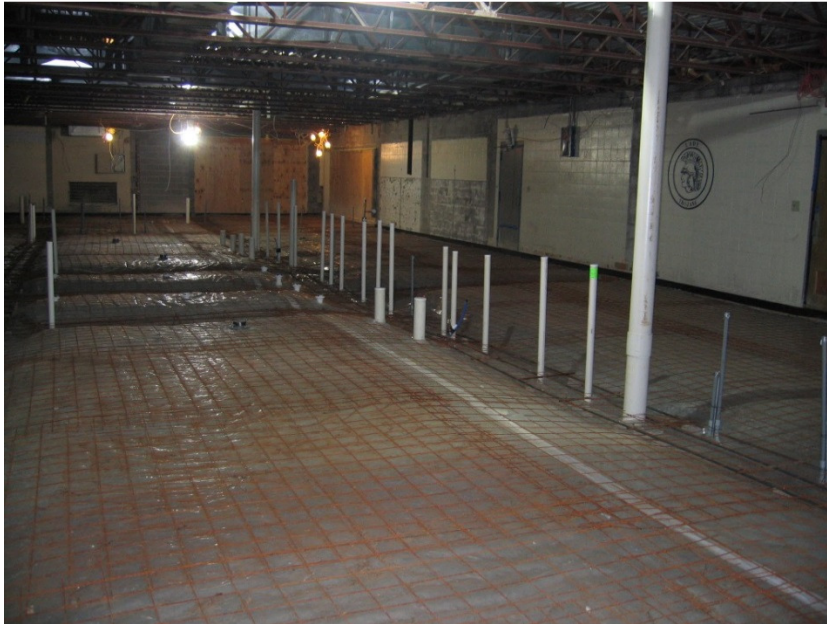
Photo 5: Below slab rough-in of electric and plumbing is complete. Vapor barrier and slab reinforcement is in place in preparation for slab pour.
