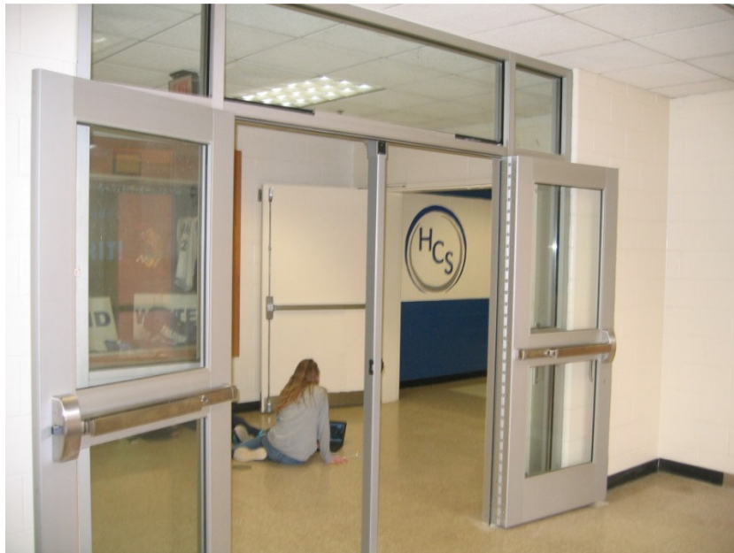
Photo 1: Storefront system and doors have been installed at the interior side of the security vestibule. SCB has requested a credit for the finish (clear anodized aluminum provide in lieu of 2 coat kynar as specified).
