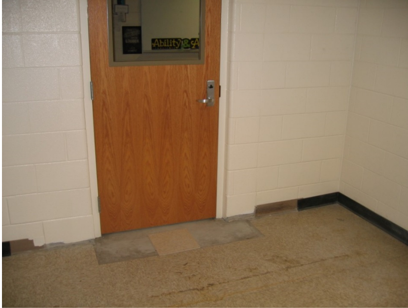
Photo 2: Flooring at vestibule will be patched to match the existing floor tile (from attic stock).
