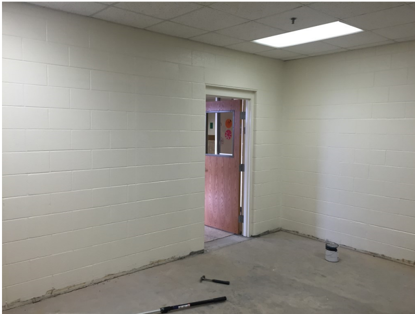
Photo 3: Existing flooring and wall base have been removed in the security office. Interior finishes are ongoing.
