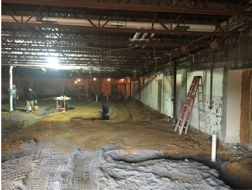
Photo 3: Interior demolition is complete within the existing locker room area (adjacent to Main Gymnasium). Below slab rough-in work is ongoing.
