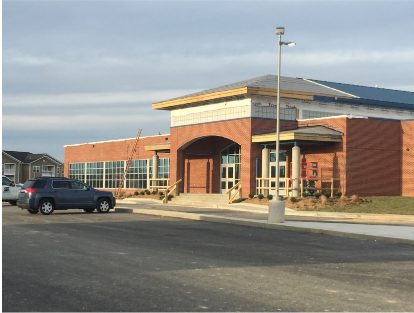
Photo 1: Metal roofing work is ongoing at the new entry lobby.
