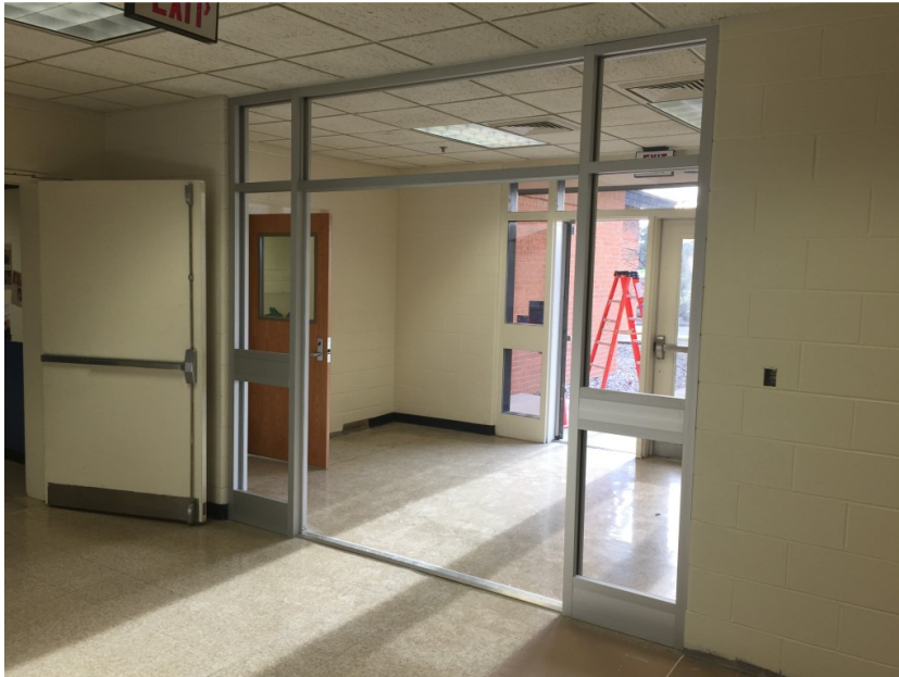
Photo 1: New masonry walls and storefront at the interior side of the new security vestibule.
