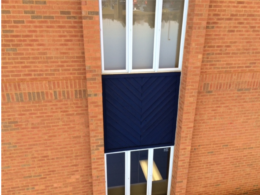
Photo 2: Completed spandrel (typical for the entire school).
