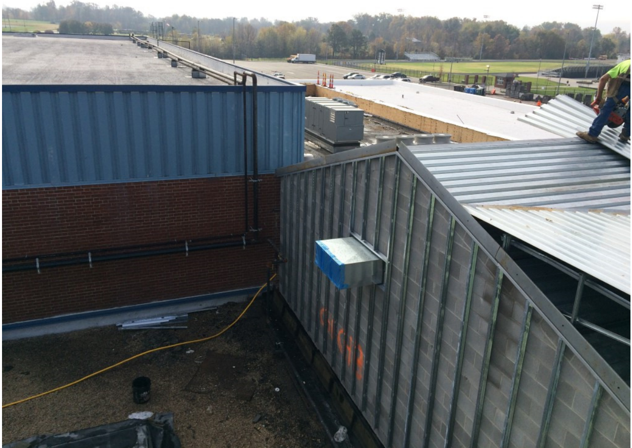
Photo 2: (Beyond) New Locker Room addition has been dried in and interior finish work is ongoing. Mechanical units above the existing locker room area have been set.
