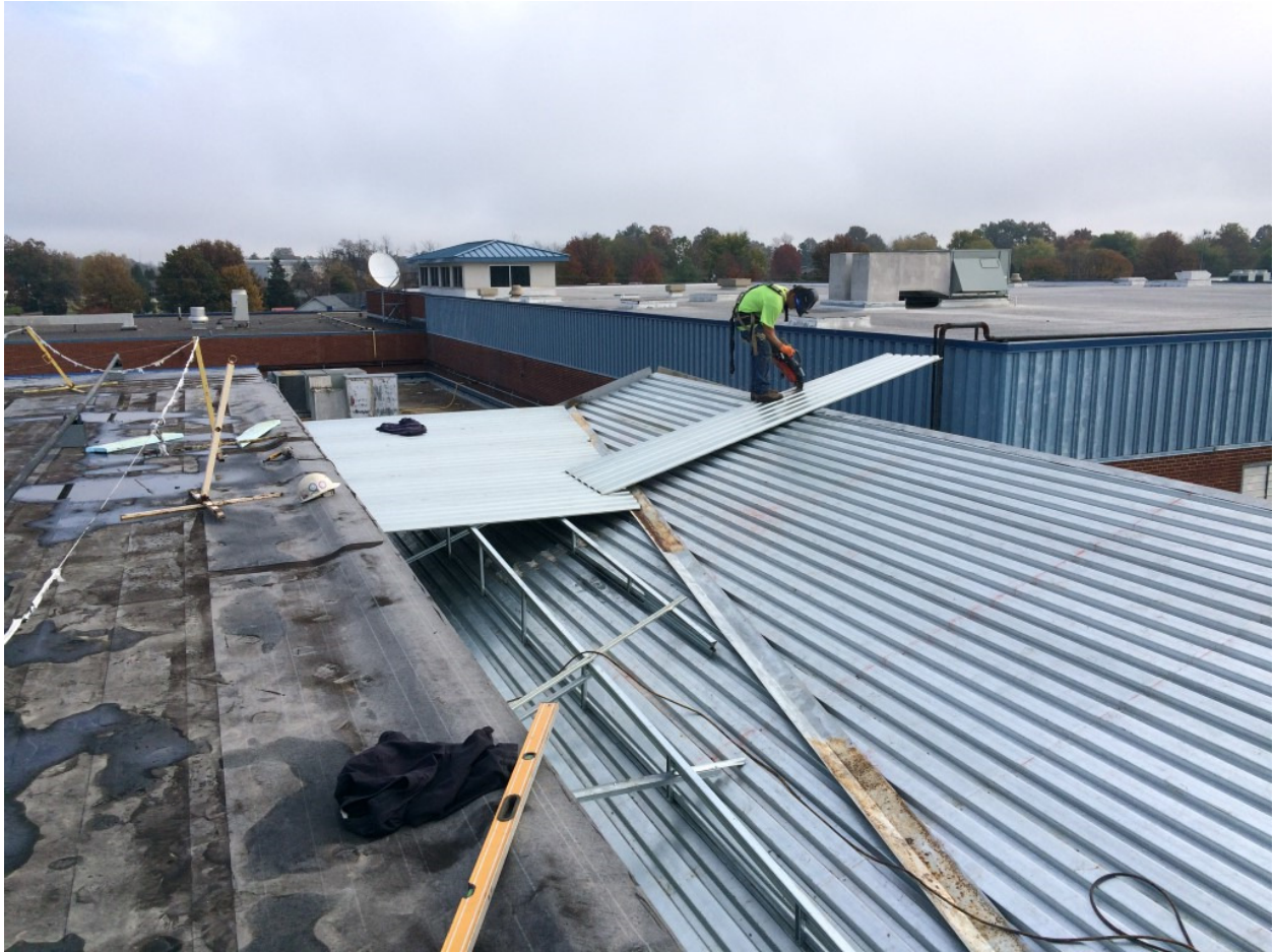
Photo 1: Roof decking installation is ongoing at the New Lobby.
