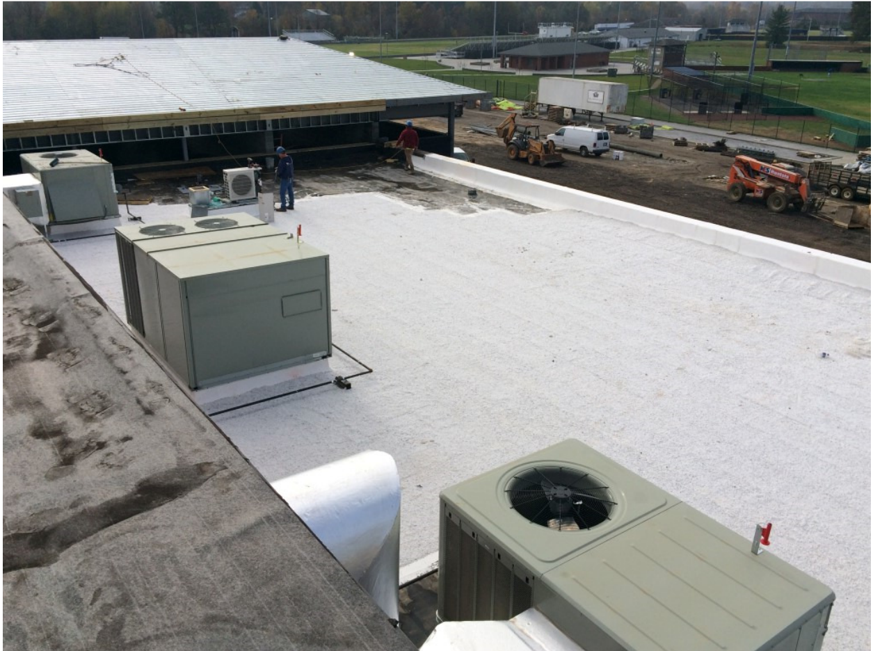
Photo 3: Wellness Center Roof is 90% complete less parapet caps and tie in to the New Lobby clerestory. (Beyond) site work continues.
