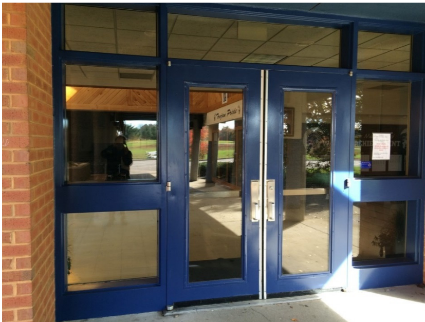
Photo 3: Exterior side of existing hollow metal doors and frames have been painted.
