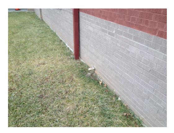
Sherman Carter Barnhart recommends adding a yard drain and redirecting the grades in this area to the yard drain to provide positive slope away from the building. Additionally, a drain to collect the condensate line is recommended to tie into the storm line.
