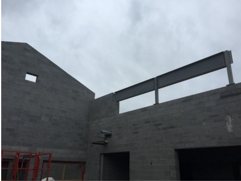
Photo 2: Steel is currently being set above the clerestory in preparation for the light gauge metal truss installation at the roof.
