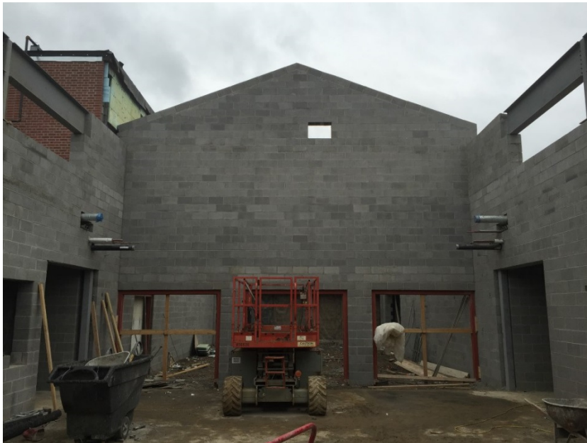
Photo 2: Steel is currently being set above the clerestory in preparation for the light gauge metal truss installation at the roof.
