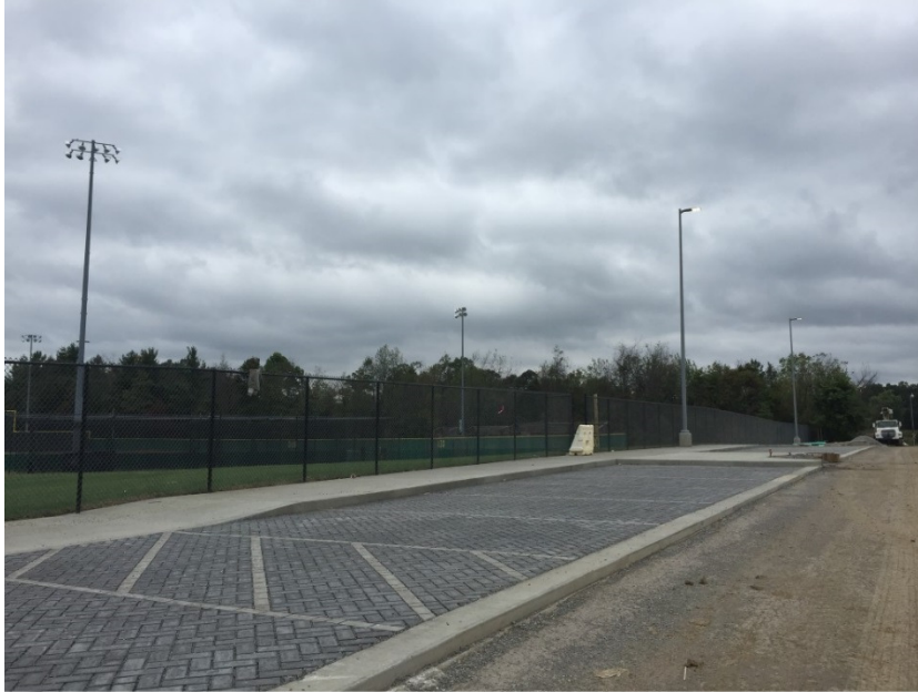
Photo 8: Permeable pavers have been installed north of the athletics complex entry.
