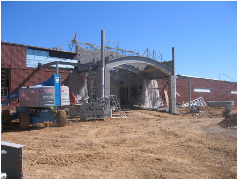
Photo 1: Masonry work and steel erection is ongoing at the new rear entry.
