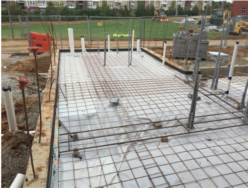
Photo 6: Below slab electric and plumbing is complete. Vapor barrier and slab reinforcement are in place and prepared for new slab at the building addition north of the existing auxiliary gymnasium.
