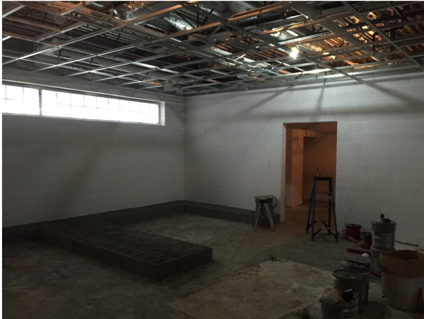
Photo 4: Rough-in work above the ceiling is nearing completion at the new locker room areas. CMU bases are being installed for the new lockers. Block filler (first coat of paint) has begun.
