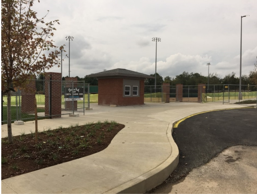
Photo 8: New Ticket Booth is in place. Morel is presently waiting for new storefront and glazing for the new ticket booth. Temporary double hung windows have been installed so that the ticket booth can be used by the school.
