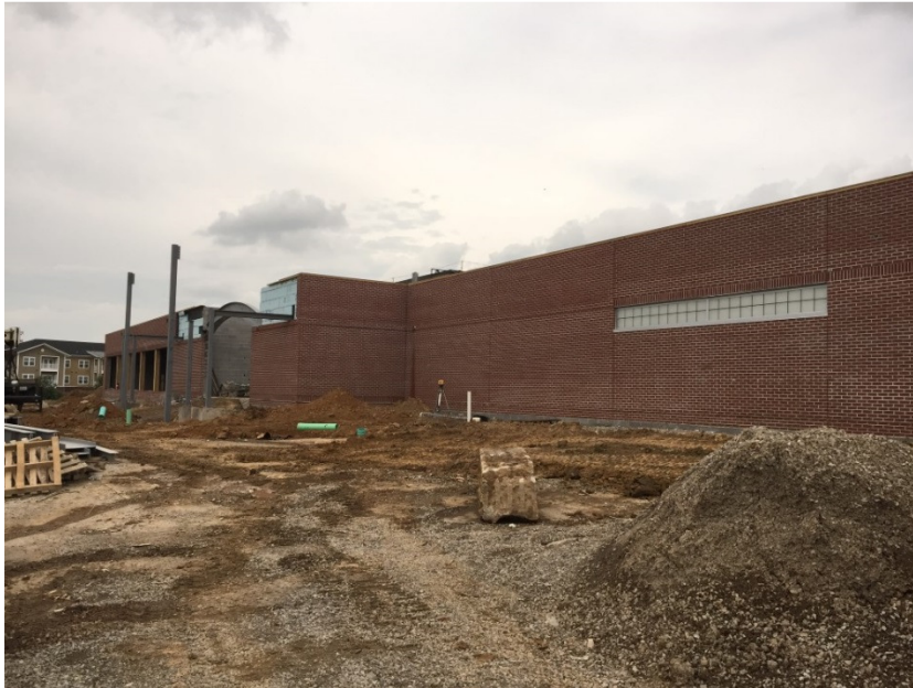
Photo 4: Exterior brick work is nearing completion at the New Locker Room addition. Exterior translucent wall panel has been installed at the locker room areas.
