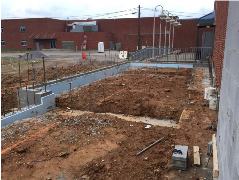
Photo 2: Footings and stem walls have been placed at the building addition north of the existing auxiliary gymnasium.
