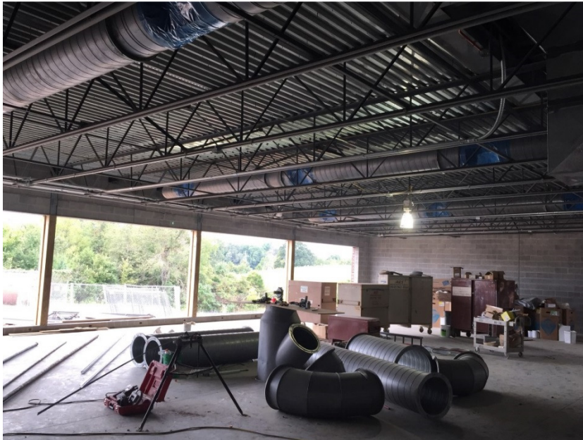
Photo 1: HVAC and electrical rough-in work is ongoing at the Wellness Center.
