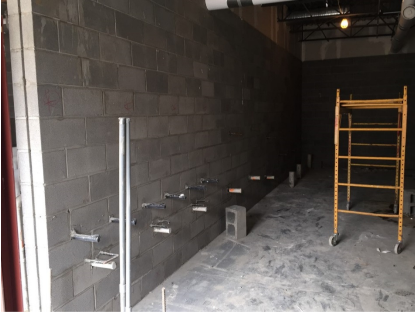
Photo 6: Plumbing rough-in work is ongoing at the New Restrooms off of the New Entry Lobby.
