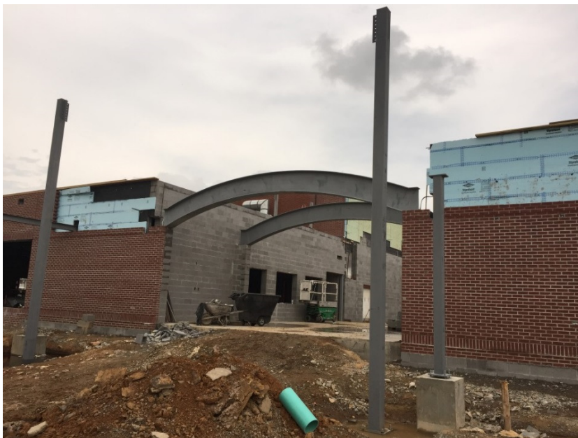
Photo 3: Structural steel is being set at the new rear entry.
