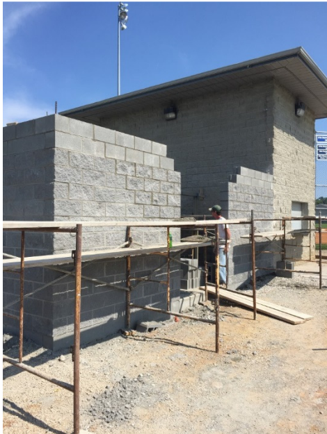
Photo 1: Exterior masonry work is presently ongoing. Truss installation is anticipated on Monday, June 8 th .
