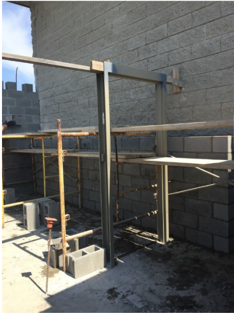
Photo 2: Interior masonry work is ongoing and hollow metal frames are being set.
