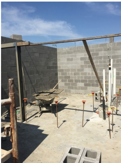
Photo 3: Plumbing rough-in is complete and slab has been placed.
