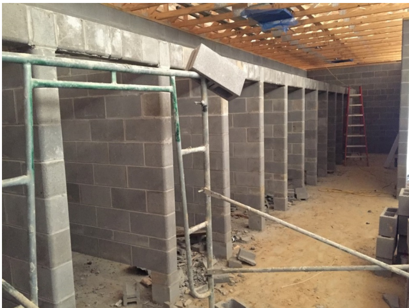
Photo 11: New toilet partitions and plumbing rough-in work is ongoing in the New Central Concessions/Restroom Building.
