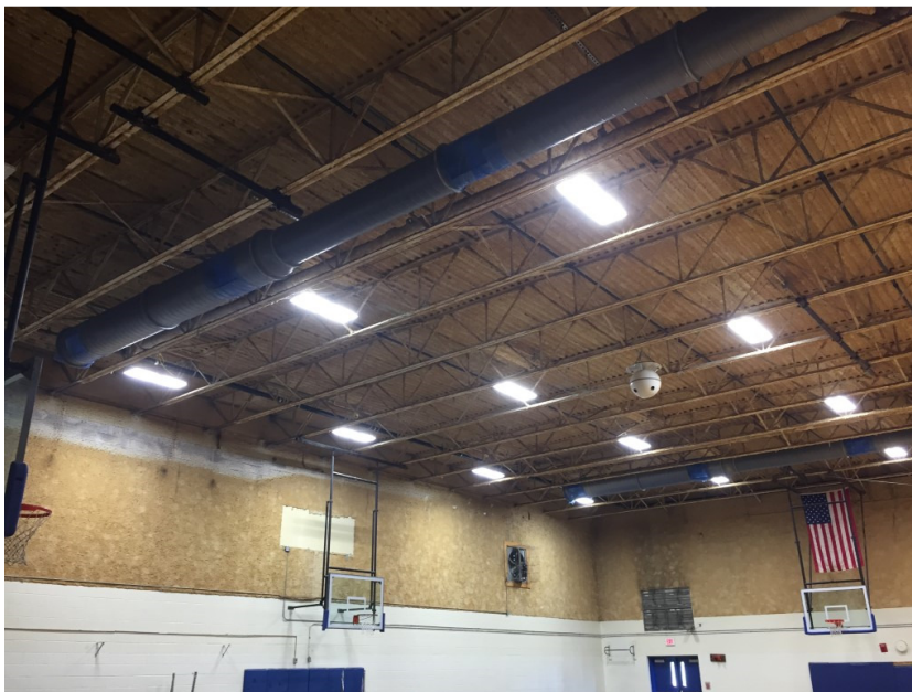
Photo 3: New ductwork and LED lighting have been installed in the auxiliary gymnasium.
