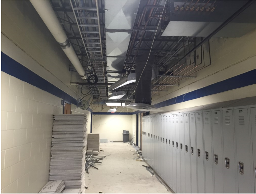
Photo 6: Demolition of existing ceiling grid/tile and HVAC rough-in is ongoing at the Freshmen Wing – Second Floor.
