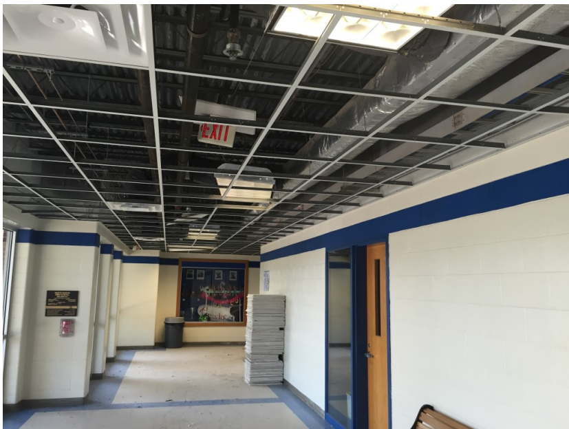
Photo 5: HVAC rough-in and ceiling grid installation is ongoing at the Freshmen Wing – First Floor.
