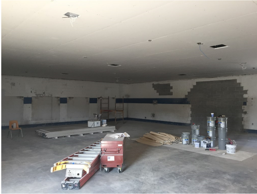
Photo 14: HVAC rough-in is complete at the new Football Locker Room area and new drywall ceilings have been installed at underside of existing wood trusses.
