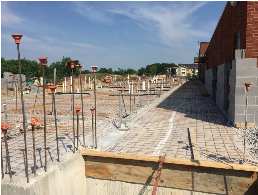
Photo 1: Under slab plumbing work is complete at the new locker room addition. Vapor barrier and slab reinforcing have been placed and prepped for slab pour on Monday, June 8 th .
