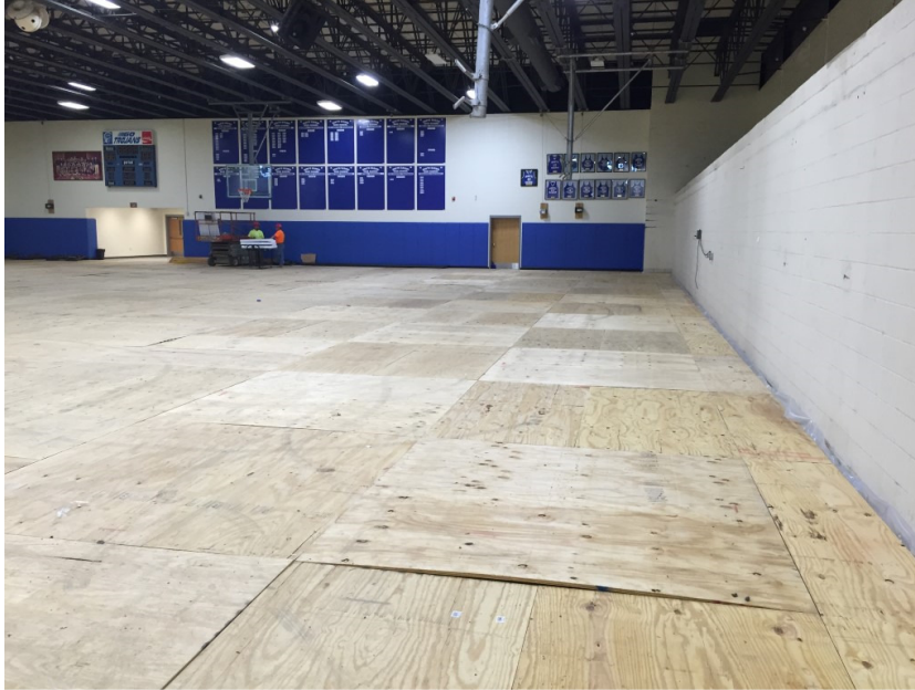
Photo 2: Construction is ongoing in the gymnasium. Plywood has been put down to protect the existing wood gym floor. Existing bleachers have been removed and walls are being prepped for new paint prior to new bleacher installation. Bleachers are presently scheduled to arrive June 22 nd . New LED gym lighting is also being installed.
