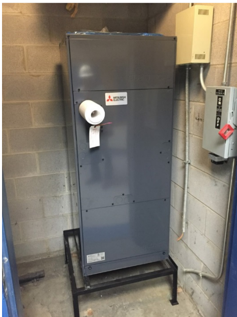
Photo 7: New mechanical units are being installed in existing mechanical closets at Freshmen Wing.
