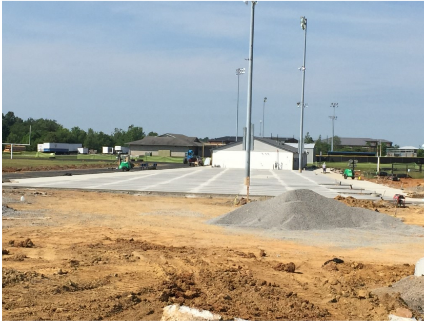
Photo 8: New foundations/slab for new home side football grandstands have been placed.
