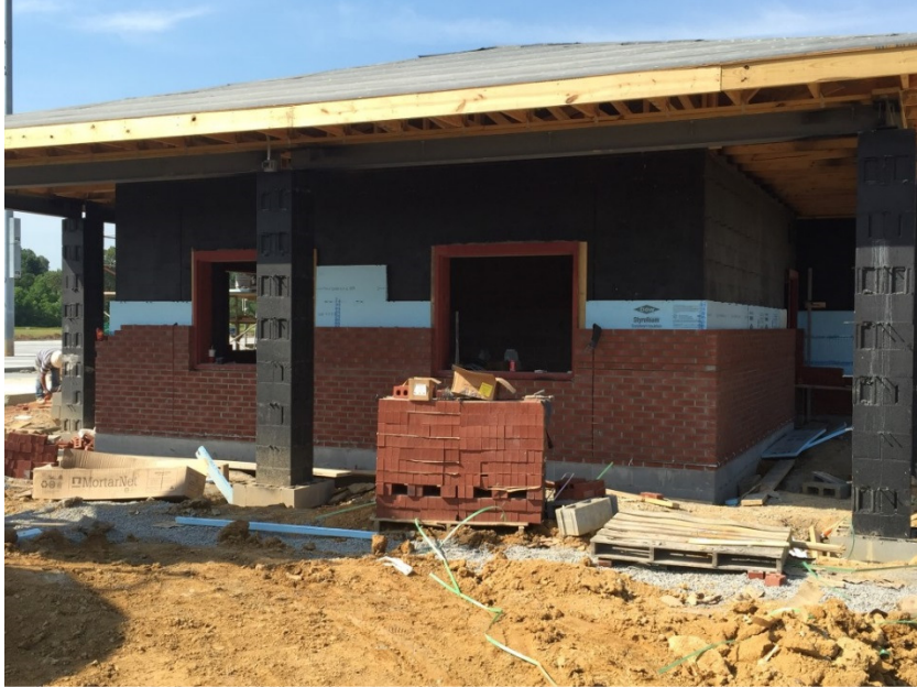
Photo 10: New cmu and dampproofing at the new Central Concessions/Restroom Building has been completed and brick work is ongoing around the perimeter of the building.
