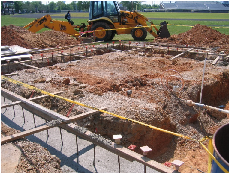
Photo 3: Footing and layout work ongoing.
