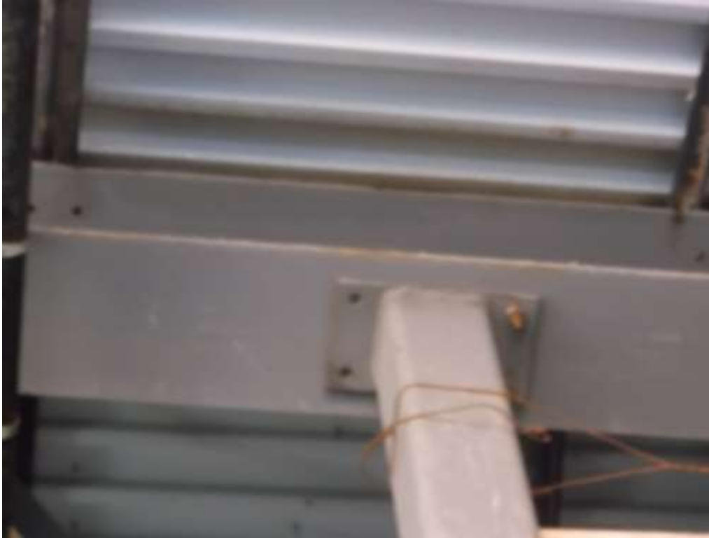
HIGH-STRENGTH BOLTS NEED TO BE INSTALLED AT COLUMN H/28
