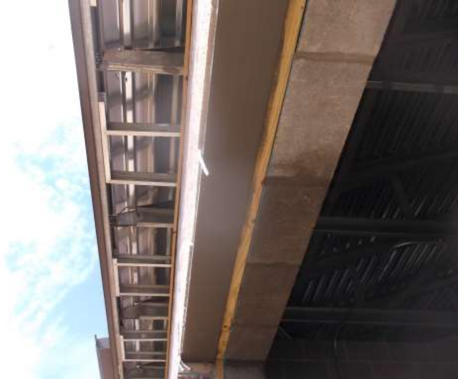
LOOSE LINTEL INSTALLED IMPROPERLY WITH LONG LEG HORIZONTAL
