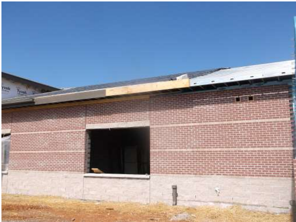
LOOSE LINTEL ABOVE WINDOW SAGING DUE TO NOT BEING INSTALLED CORRECTLY
