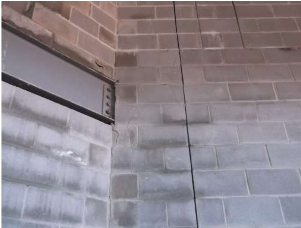
CMU FROZE AND CRACKED AT COLUMN F/26
