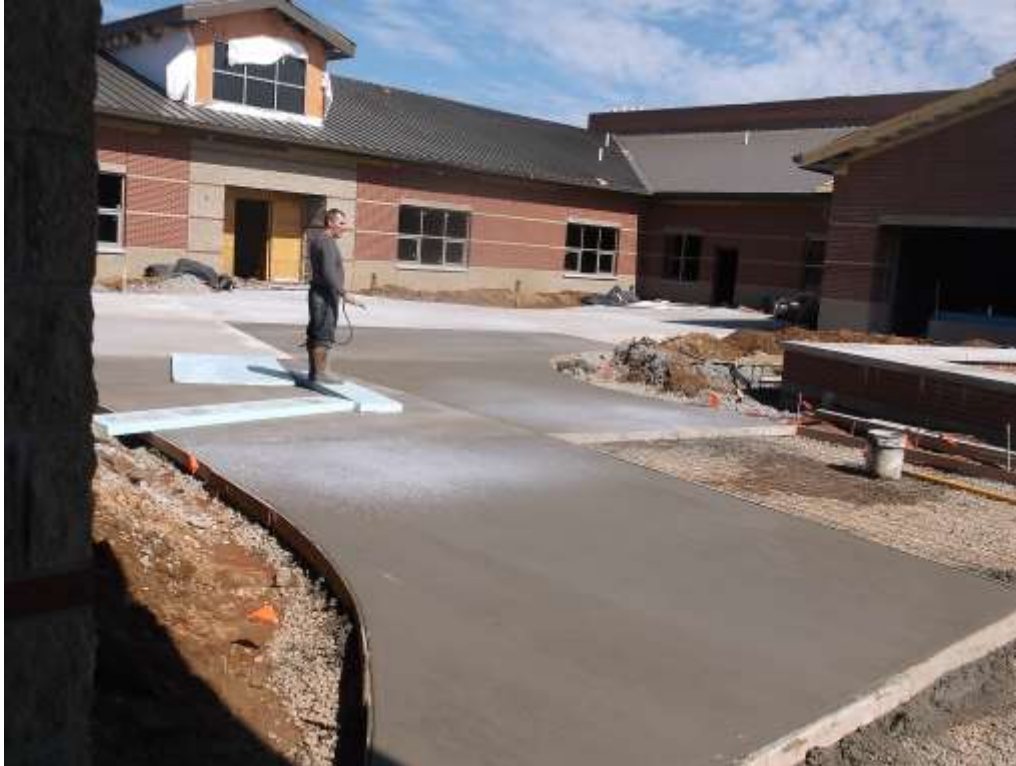
COURTYARD CONCRETE IS BEING INSTALLED
