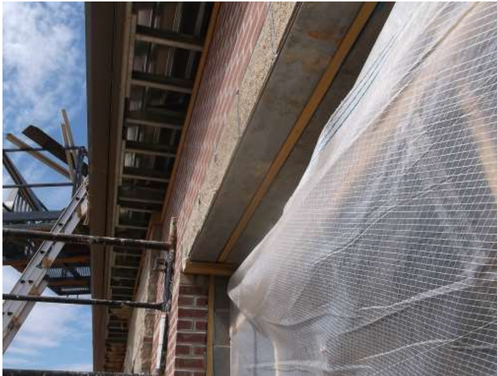
LOOSE LINTEL TO BE INSTALLED (LLV) LONG LEG VERTICAL NOT HORIZONTAL
