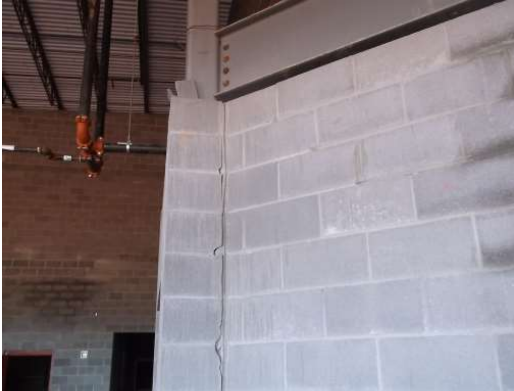
CMU FROZE AND CRACKED AT COLUMN H/28
