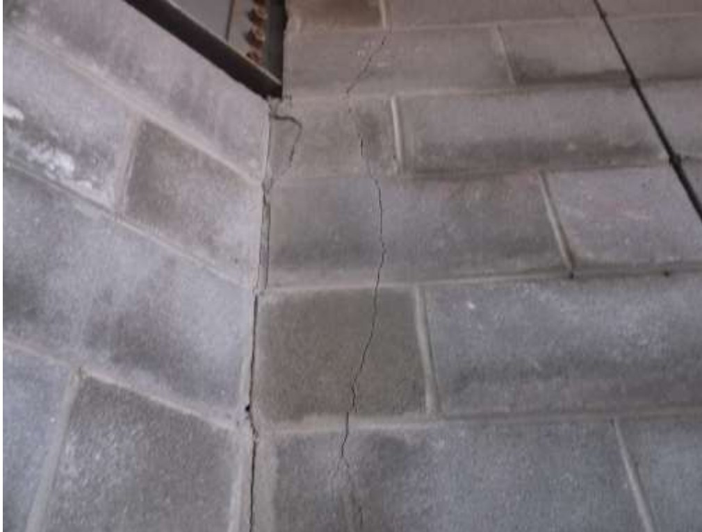
DAMAGED MASONRY AT COLUMN F/26
