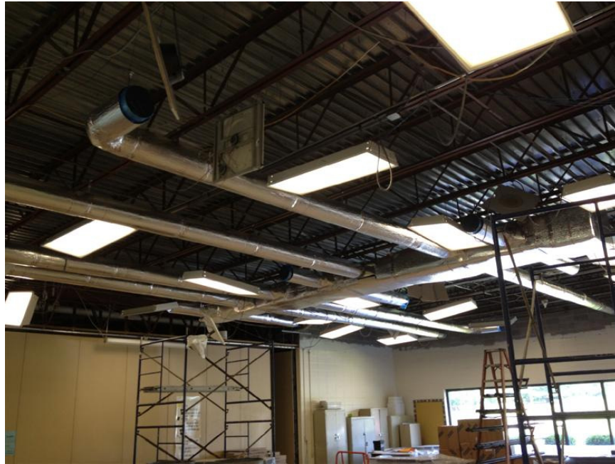
New ductwork in Existing Cafeteria
