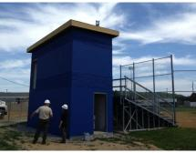
5. Football Press Box masonry and paint is complete. Wood framing is ongoing. Bleacher installation is near complete. Bleacher railing and chain link fence installation is underway. Stairs connecting bleachers and Press Box are forthcoming, pending Press Box porches and stair material delivery. Overhead coiling counter top doors have been installed.
