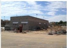
2. Field House Exterior masonry openings are being prepared. Solid masonry sills are being made on site. Masonry installed at door jambs appears thin compared to jamb detail drawing. Contractor to verify frame is adequately anchored and masonry provides full thickness for spray foam insulation stop. Further discussion is required for these doors before face brick is installed.
