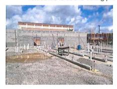
3. Masonry installation at beam between Cardio and Weight rooms was reviewed by mason and RTA on site. Installation was acceptable and no change is required at window head as installed.
