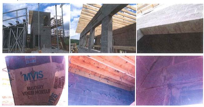
10. Football Press Box column bases and columns have been installed. Additional testing of the footings may be required. Surface hardness of top of footing was demonstrated by multiple hammer strikes.
