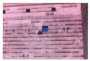
5. Masonry door heads were reviewed at Cardio and Weight room. Mortar joints were found excessive and future door frame installations are to be done more carefully. Contractor stated sealant installation would minimize visual impact of wide mortar joint. No new action is required at this time.
