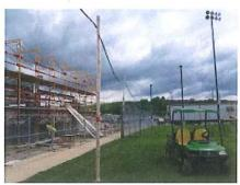
7. Softball press box masonry and wood framing is complete. Block fill and painting are to begin shortly. Grout or mortar was observed on the face of the CMU. Care is to be taken with cleaning CMU and block fill placement to insure excess grout or mortar does not telegraph through the finish paint.
