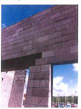
4. Openings in masonry walls for mechanical ducting were discussed at the Cardio room. Contractor is to verify elevation does not conflict with bond beams for upper and lower roof as well as finish ceiling heights. Preliminary indications in the field are that all items have been considered and installed correctly.
