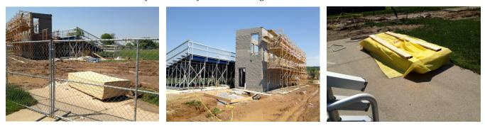
5. Excess grout was observed on both Press Box buildings. Care is to be taken during cleaning to remove grout. CMU is to be painted and excess grout in the pourous surface may telegraph through the finish.
