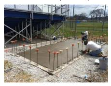
3. The concession building footers were complete and grading was at subgrade level. The 57 stone shown in the picture will be capped with 4" of DGA under the building pad per Ken Jones. It was discussed that if any utilities are in the zone of influence they should be backfilled with flowable fill.
