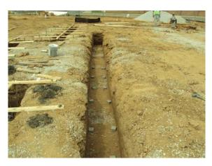
2. The continuous bars and dowels within footing sections scheduled for concrete today were reviewed. The bars were properly supported and the reinforcing steel was tied and secure. CSI is performing all required testing and special inspections. Special Inspector, Daniel Huffaker, was on site this date. He said that the reinforcing steel placed thus far was installed as indicated in the structural drawings. No deviations had been reported.
