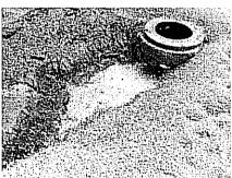
3. Building pad is still under construction as of this observation. Photos illustrate current work. The existing drywell is still to be abandoned and removed/filled.
