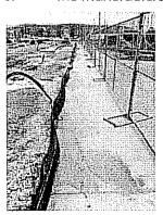
7. The silt fence along the pedestrian path is stretching and showing minimal failure. Contractor should address the cleaning of the sidewalk periodically and as needed.
