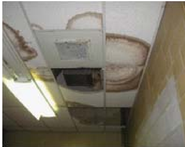
Damaged ceiling tile from a leaking roof at Fern Creek High School.
