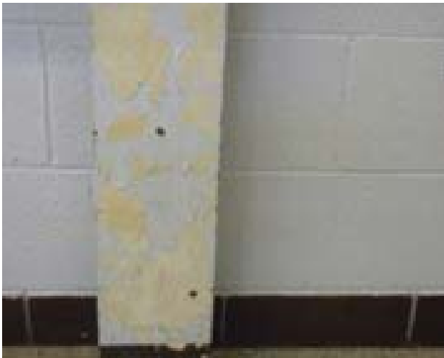
Peeling paint at Dixie Elementary, a school with a large population of special needs students who were reported to have eaten some the peeling paint (which tested positive for containing lead).
