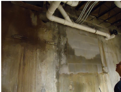
The existing concrete walls adjacent to the coal chute also show signs of water infiltration. These surfaces were “wet” to the touch.
