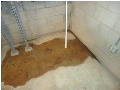
Across the room from exterior wall of the coal chute, standing water was noted at the southeast corner of Storage Room 002. Upon closer investigation, it appeared that water infiltration was occurring from under the existing concrete slab – hydrostatic pressure.
