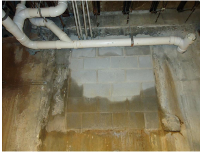
Water infiltration through sealed existing coal chute. The area of saturation of the coal chute is approximately 3-5 feet below exterior grade. The coal chute is located in Storage Room 002.
