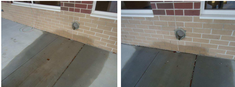
Water flowing from overflow scupper located at south elevation, to left of exterior Cafeteria entrance.
