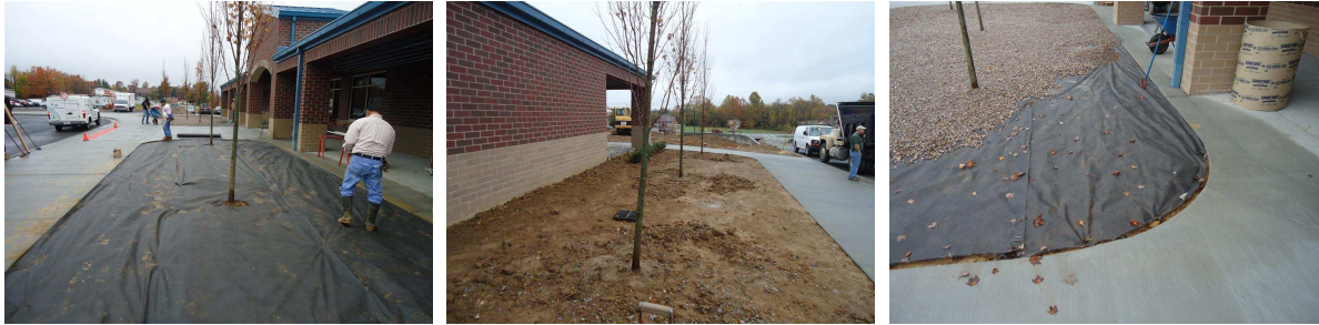
Installation of pea gravel and landscaping has started at islands along south of building, Cafeteria entrance.
