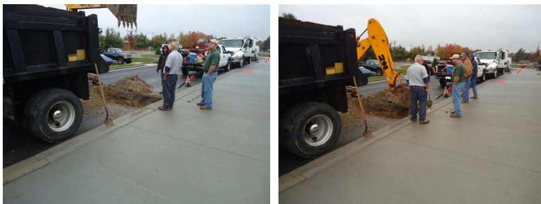
Site contractors removing area of car loop and drive to investigate damaged existing sanitary sewer pipe.
