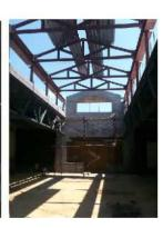
The structural steel joist girders, beams, and roof trusses have been installed within the Cafeteria at the new clerestory roof area. Metal roof decking has been installed on the lower sloped roof areas and roof deck installation has started on the clerestory.
