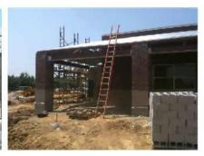
The structural steel framing at the south walkway covers in front of the Cafeteria entrance has been installed along with the light gauge metal trusses. At the front of the building (east) some metal roof decking has been installed.
