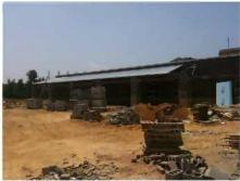
Ongoing masonry work at the front main entrance masonry portico. Contractor is awaiting delivery of steel rolled beams at portico.
