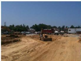
Per American Engineers (geotechnical engineer), highly organic soils have been encountered at the south area of the site, in front of the Cafeteria entrance. A new car loop and parking lot will be provided in this area. The highly organic soils are unsuitable for paving. Therefore, they must be undercut, removed, and approved structural fill material must be placed in these areas.
