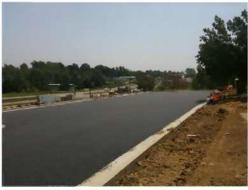
Portion of north and west loop around the Gymnasium has been paved. Curb and gutter installation has been completed in these areas.
