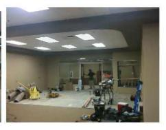
Media Center work will be completed by start of school, Wednesday, August 3. Carpet installation is almost complete. Media Center furniture was being delivered and installed in space. Above-ceiling punchlist was conducted by STW the week prior so that suspended ceiling installation could be completed.
