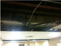
New interior brick masonry in front Lobby 100 has been installed. New soffit work will be constructed in order to lower suspended ceiling height at rear of Lobby 100 to accommodate low height of existing masonry walls and plumbing items above.
