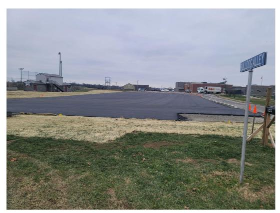
The new parking lot on the main campus had the base layer of asphalt added and will have lines striped soon.
