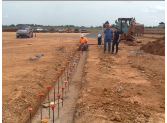
Photo # 4 - Exterior Wall Foundation
