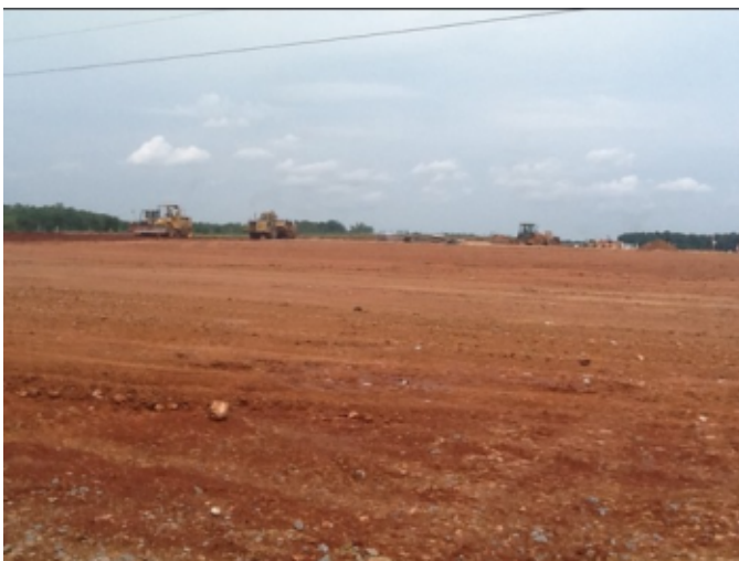
Photo # 1 - Site Grading
