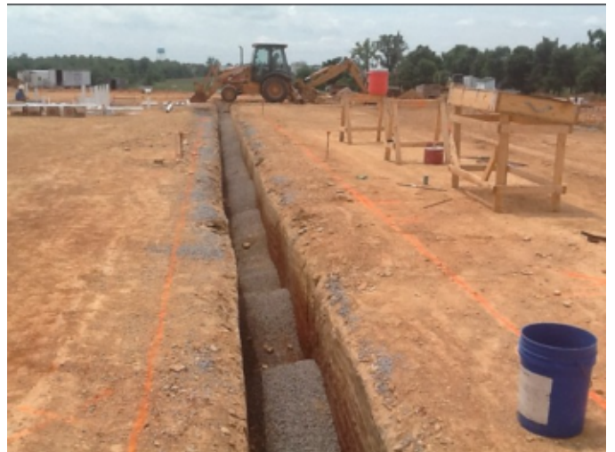
Photo # 12 - Ditch for Plumbing
