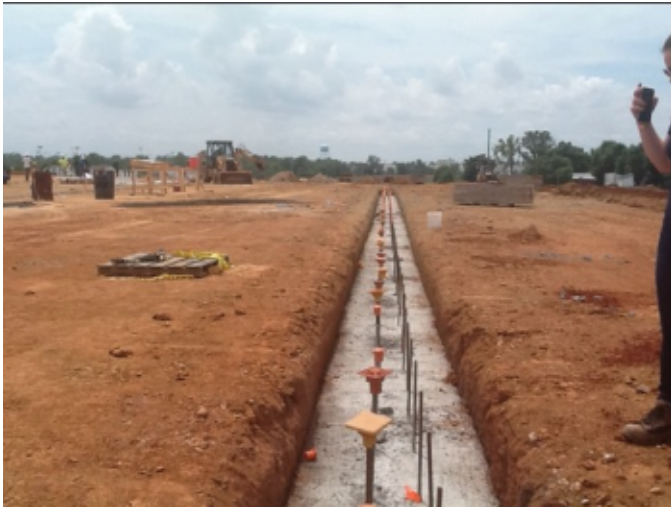
Photo # 26 - Exterior Wall Foundation adjacent to Bus Loop
