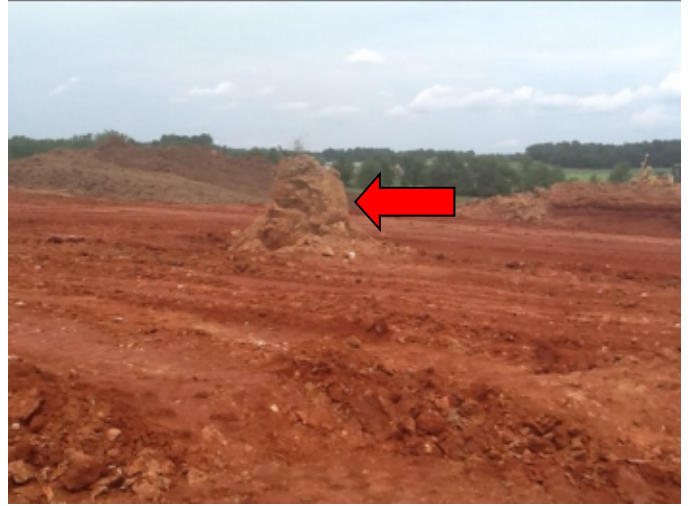
Photo # 21 – Geothermal Test Well # 1
