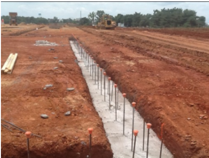
Photo # 24 - Rear Exterior Foundation
