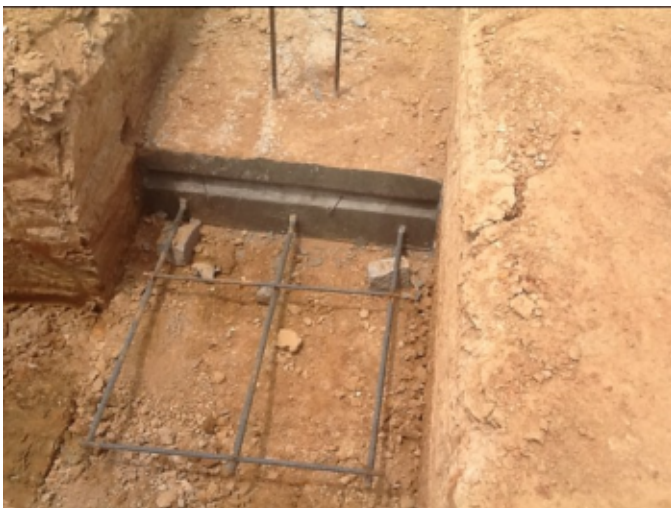
Photo # 5 - Rebar Extended
