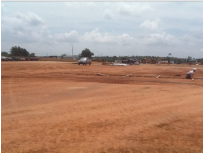
Photo # 14 - Building Pad
