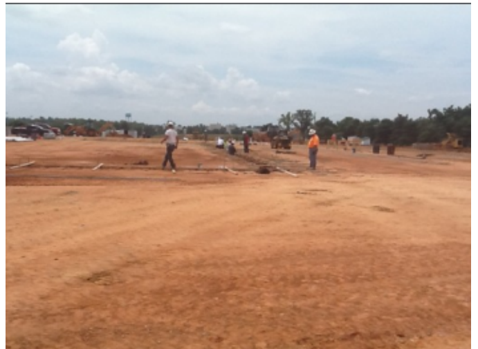
Photo # 13 - Building Pad
