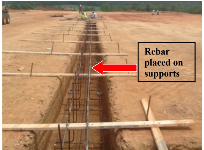
Photo # 6 - Foundation prior to placement of Concrete
