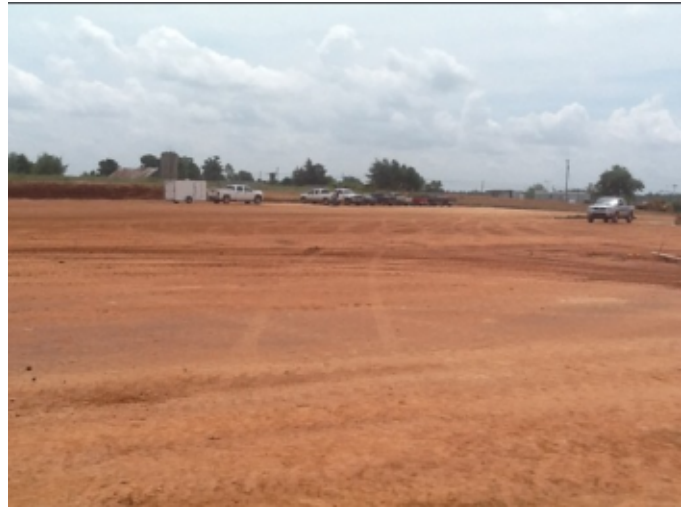
Photo # 15 - Building pad
