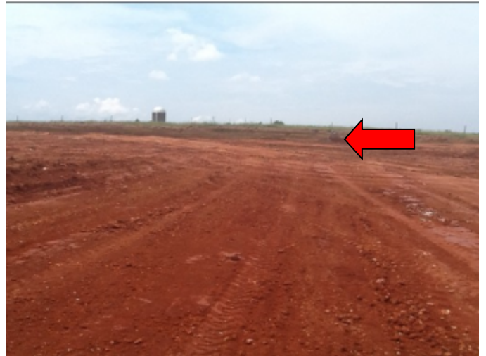
Photo # 23 - Geothermal Test Well #2
