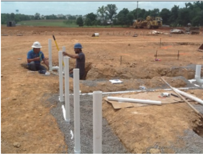
Photo # 9 - Rough In Plumbing
