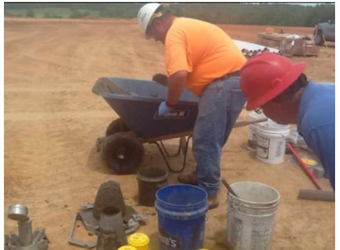
Photo # 29 - Special Inspection Testing
