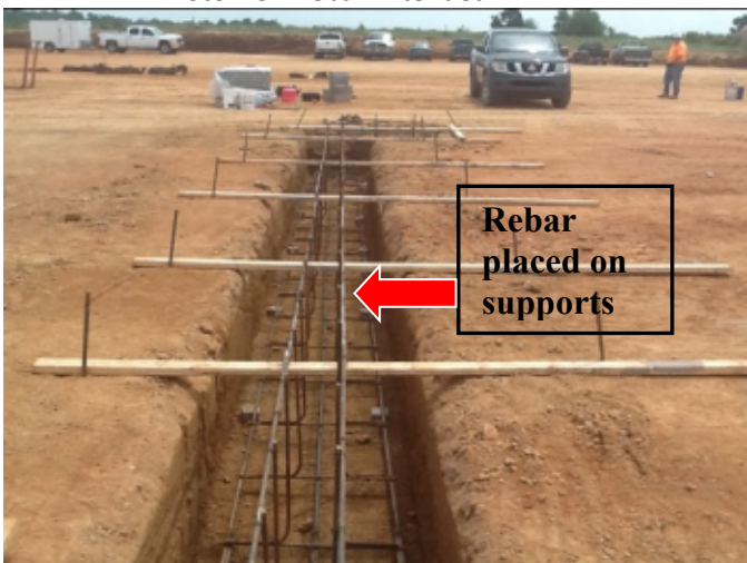
Photo # 7 - Foundation prior to placement of Concrete
