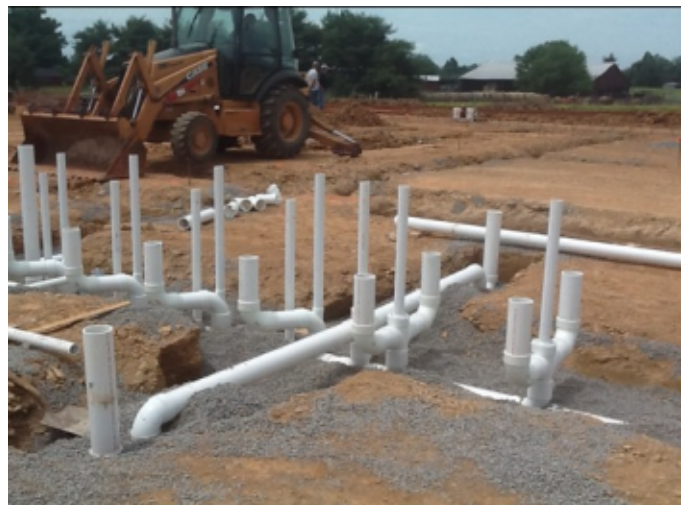
Photo # 8 - Rough In Plumbing
