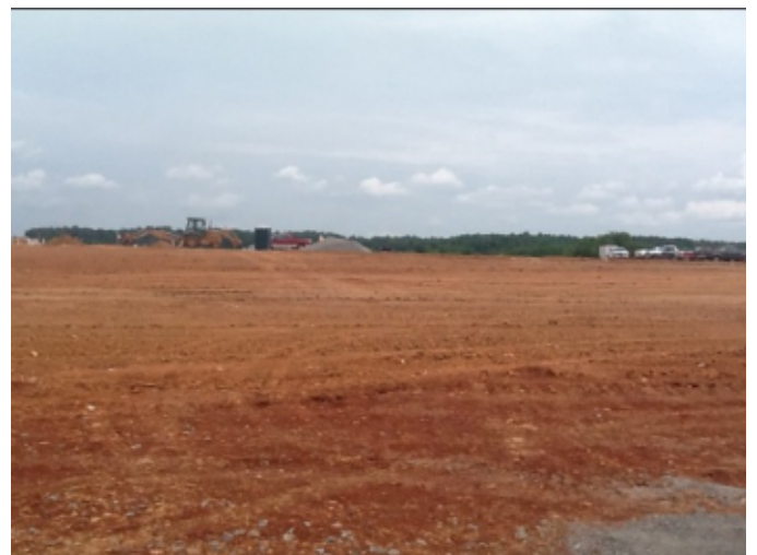
Photo # 2- Site Grading
