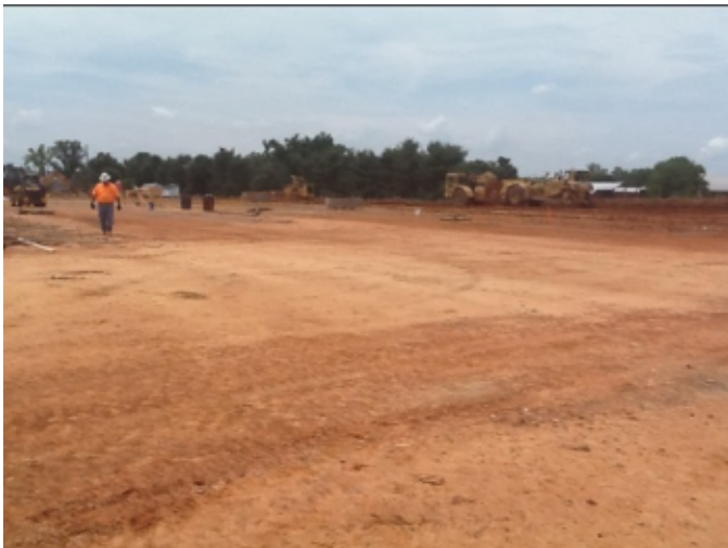
Photo # 12 - Building Pad
