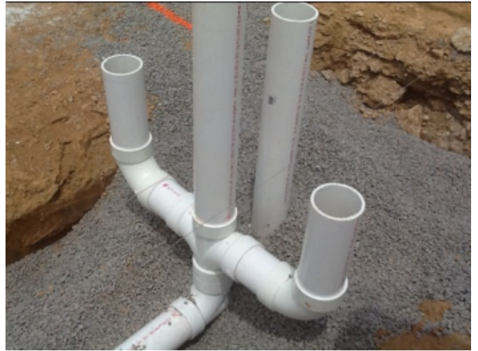
Photo # 10 - Rough In Plumbing
