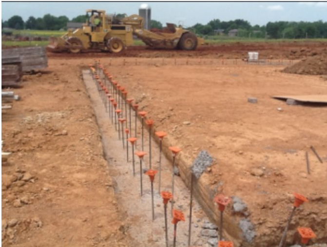
Photo # 3 - Exterior Wall Foundation
